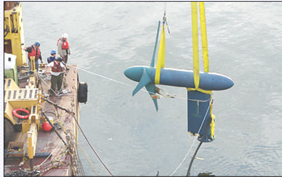
In this 2006 photo, a Verdant Power turbine is lowered into the river off Roosevelt Island. (Associated Press)
