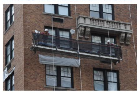
The Department has identified the use of a stand-off bracket as a contributing factor in recent suspended scaffolding incidents, and has banned their installation and use in NYC. If a suspended scaffold currently has a stand-off bracket installed, the
