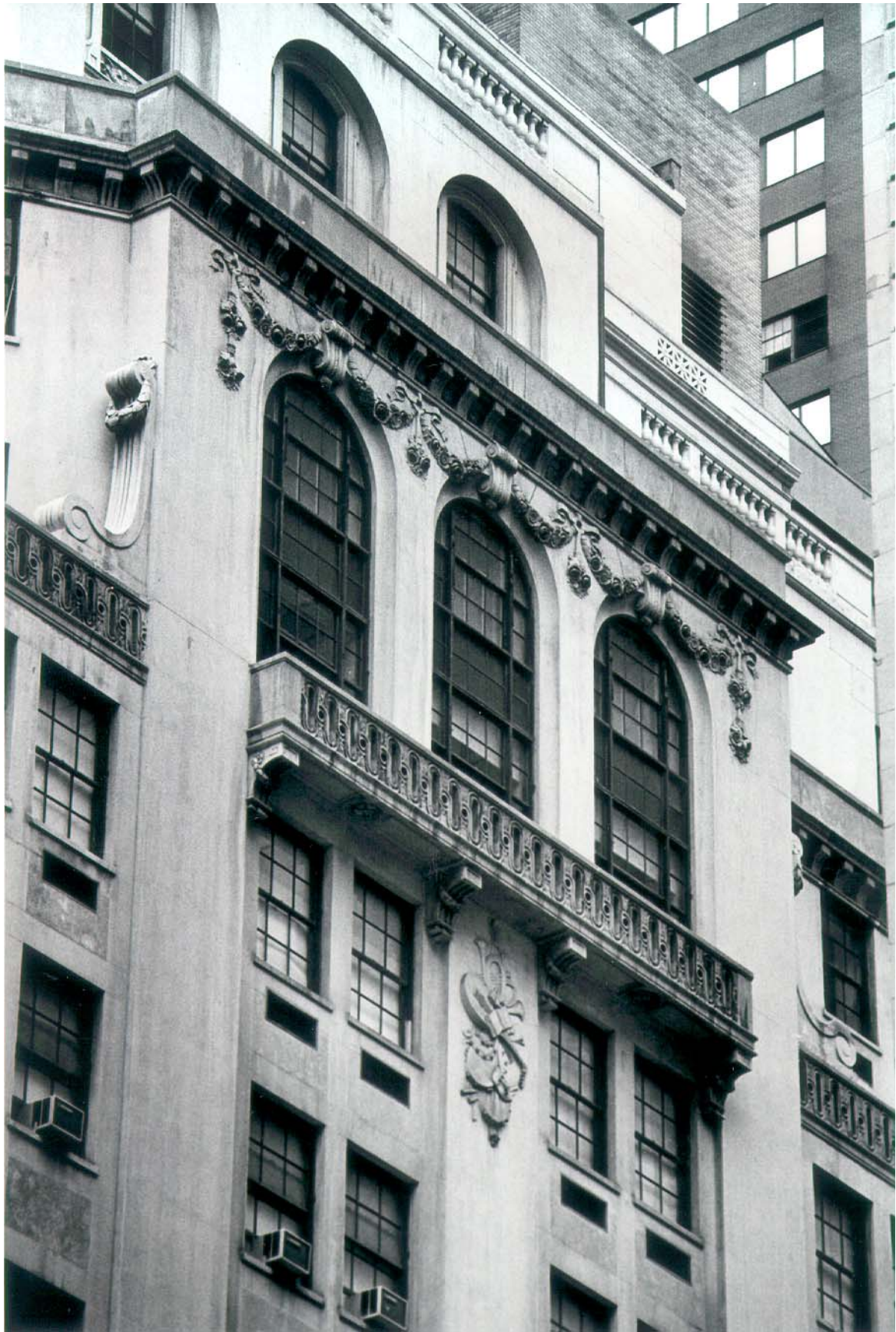
Aeolian Building (later Elizabeth Arden Building), detail of East 54 th Street facade Photo: Carl Forster
