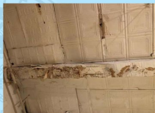
Pictured: Water Damage and Rust
