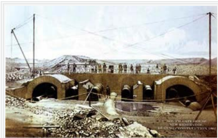
South Gate House New Reservoir, during construction 1862.
