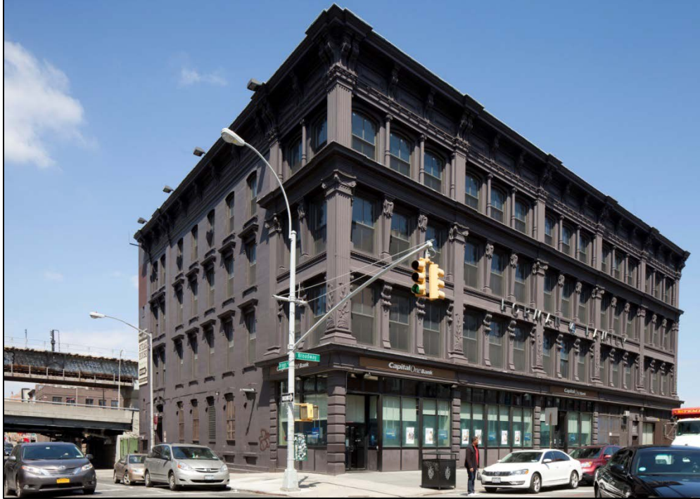
183-195 Broadway (aka 833-843 Driggs Avenue) Borough of Brooklyn, Tax Map Block 2446, Lot 51 Photo: Landmarks Preservation Commission, 2014
