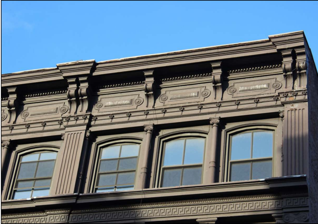
183-195 Broadway Upper Story and Cornice Detail Photo: Corinne Engelbert, 2015
