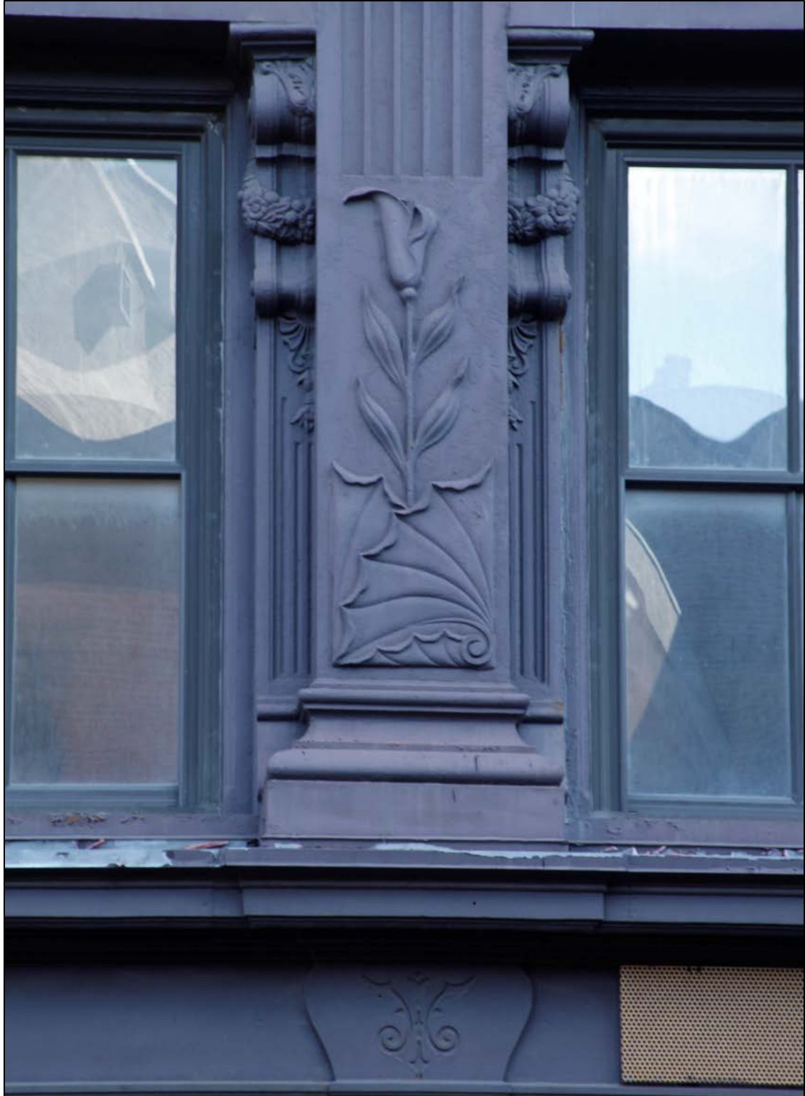
183-195 Broadway Facade Detail Photo: Sarah Moses, 2016
