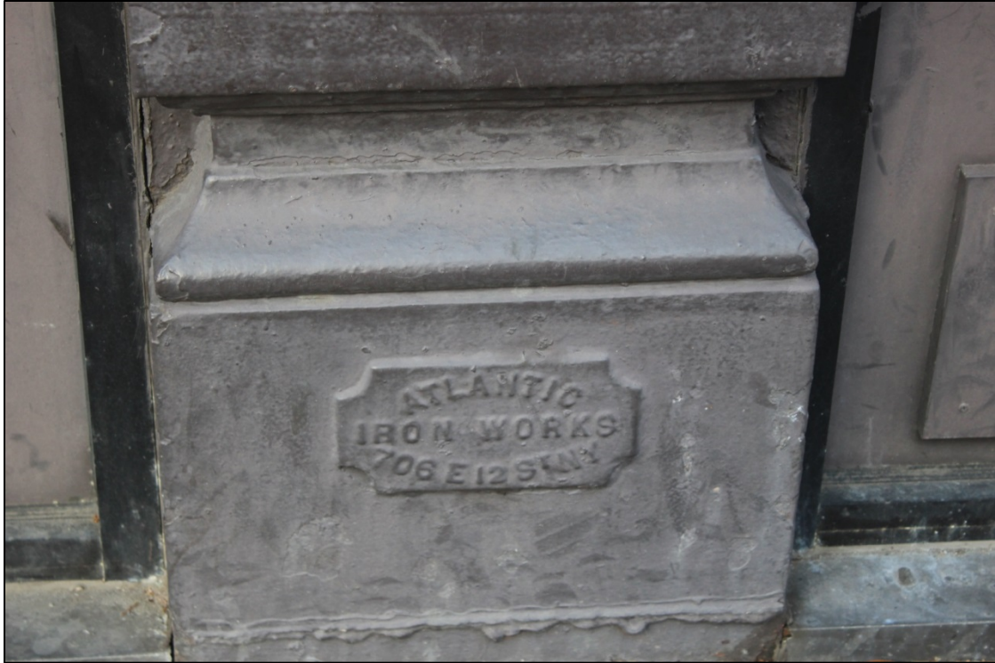
183-195 Broadway Foundry Mark Photo: Corinne Engelbert, 2015
