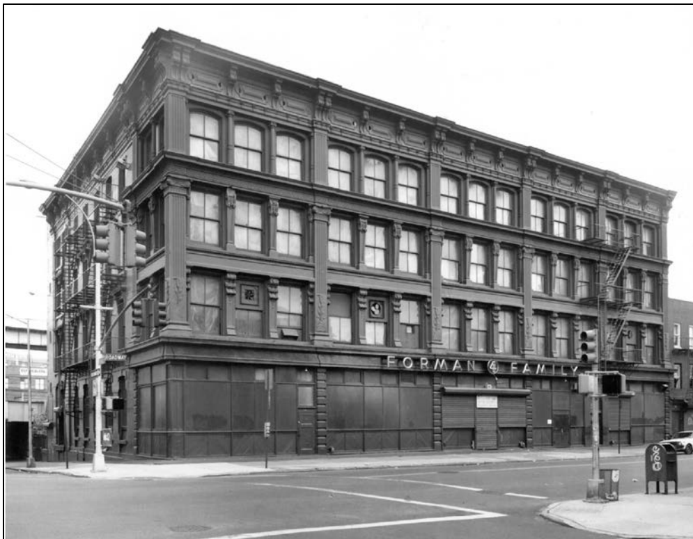
183-195 Broadway Source: Friends of Cast Iron Architecture Photo: Peter M. Lerman, July 1990
