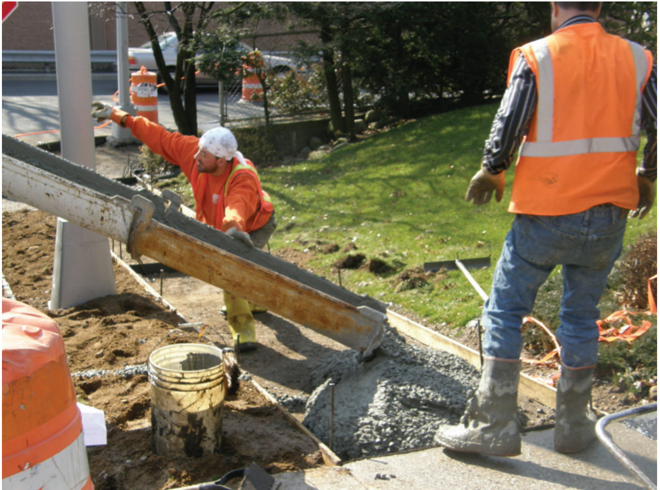
Workers pour cement during sidewalk reconstruction.
