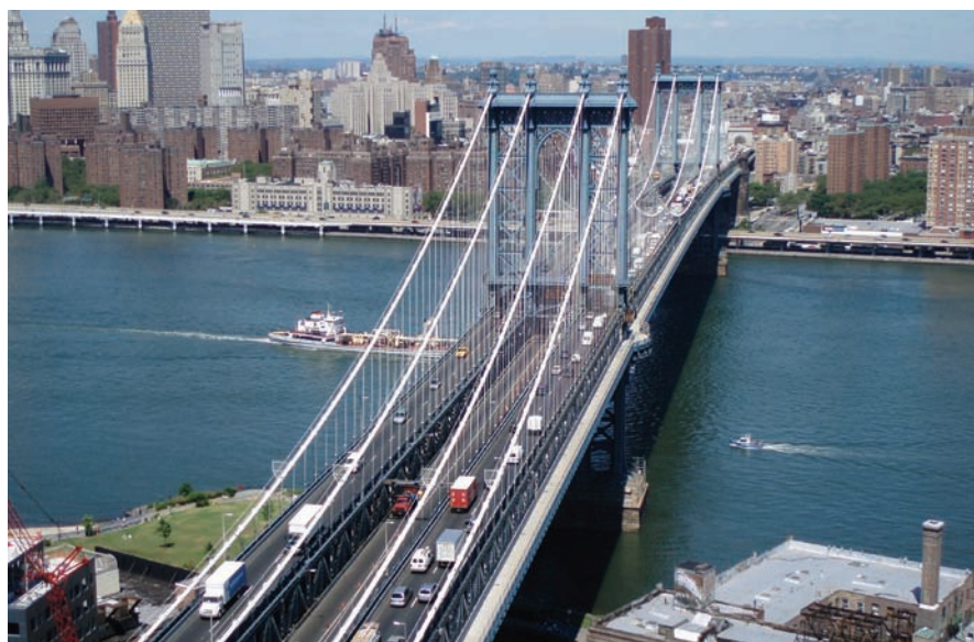
Permit applications near bridges are subject to approval by the Division of Bridges.
