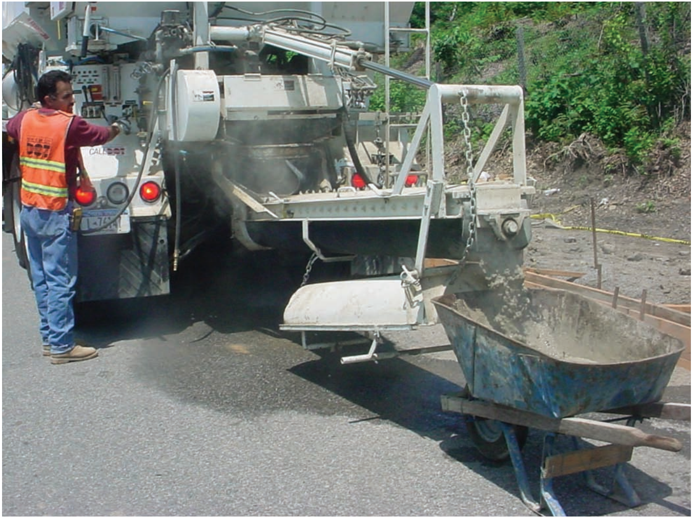
All work within the street requires a NYC DOT permit to minimize construction impacts.
