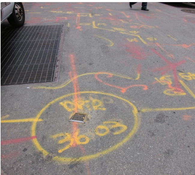
Streets can hide a complex infrastructure of underground utilities. One call to New York 811 provides for where gas (yellow), electric (red) and phone (orange) are located.
