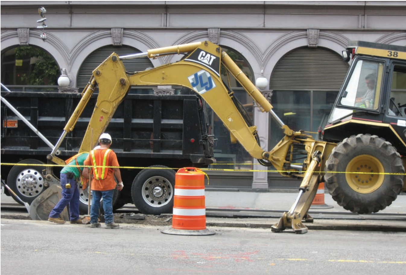
Street work at Third Avenue and Saint Marks Place, Manhattan as part of a larger Cooper Square area reconstruction project.
