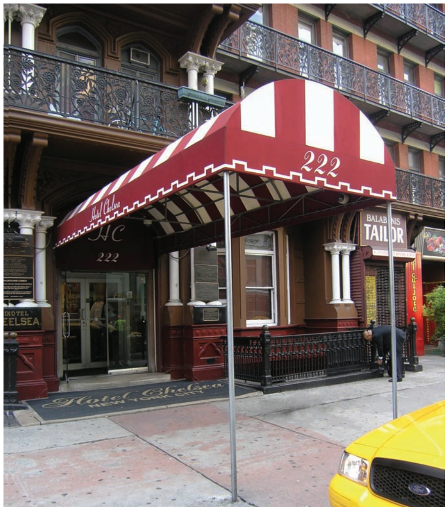
NYC DOT authorization is required before installing a canopy over the sidewalk.
