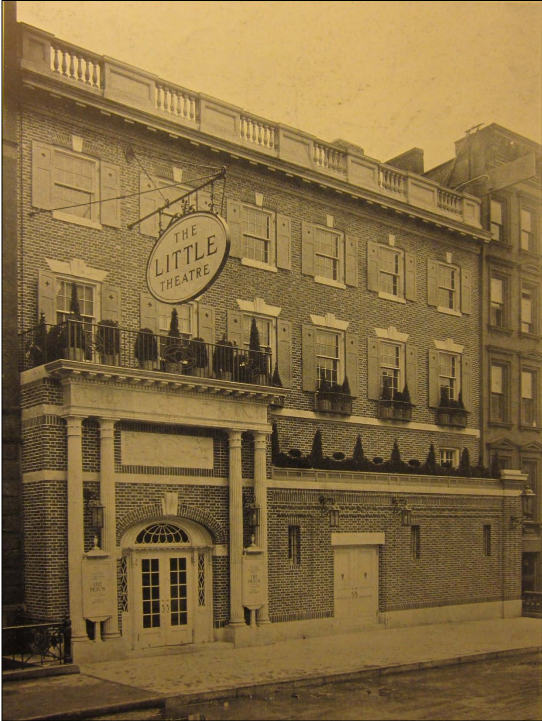
The Little Theatre (now Helen Hayes Theatre) 240 West 44 th Street, Manhattan Source: The Brickbuilder (1912)
