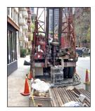
Now: DEP faces the same challenges working with tight spaces when drilling for core samples for City Water Tunnel No. 3. 2/26/2003
