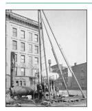
I ben: Drill machine rigged to take rock core samples in preparation for City Water Tunnel No. 1 construction in Upper Manhattan. Challenges included using tons of explosives to blast tunnel in heavily populated neighborhoods, disposing millions of tons of debris and avoiding interference with subway and sewer lines. 10/13/1909
