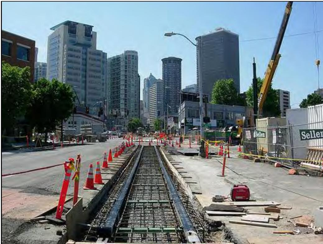
As reported in the *Seattle Streetcar Network Feasibility Study*, constructing a streetcar network in Seattle was expected to be similar to the construction of peer city streetcar lines, particularly Portland. In the typical construction method for the streetcar track system, the top 12 to 18 inches of pavement is removed and replaced with rail-embedded reinforced concrete slabs within a trench
