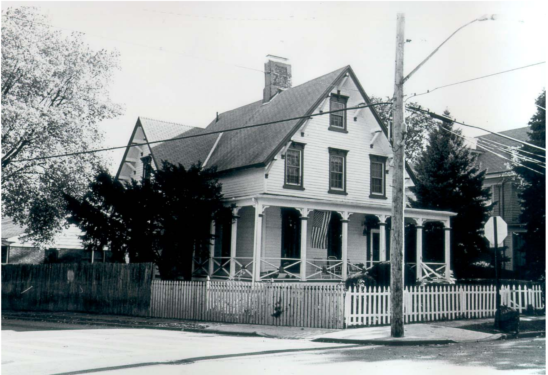
View from the northwest showing the Heberton Avenue and Bennett Street facades Photo: Carl Forster
