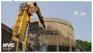
esterday, work got underway to demolish a tank along the East River that was used to store sludge from the Newtown Creek Wastewater Treatment Plant until it could be loaded onto boats and removed to one of DEP's dewatering facilities. DEP's
