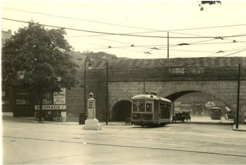
Burnside Avenue Bridge, Removed Lehman College Archives, 1920
