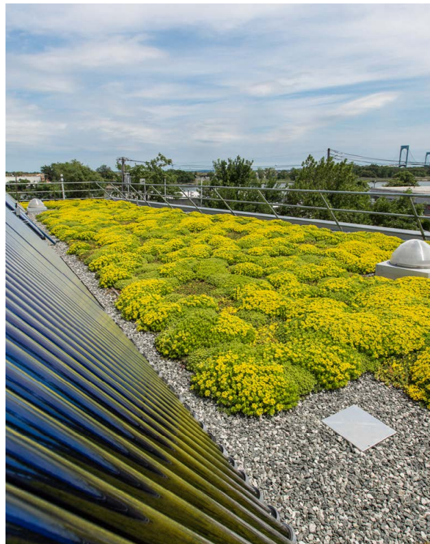
Green Roof at Zerega EMS Station
