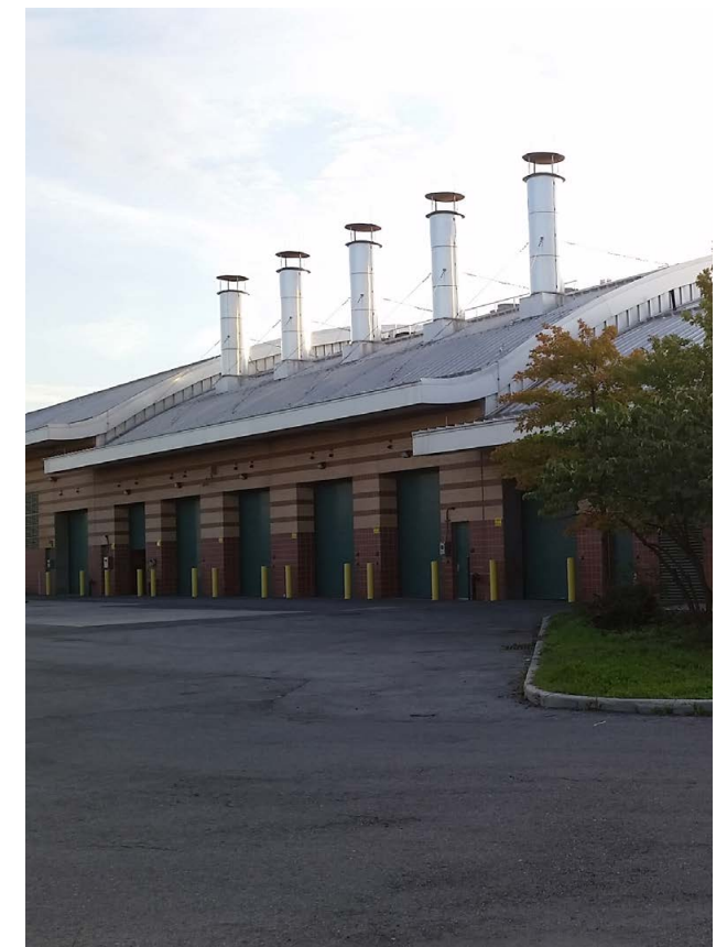
Paerdegat Basin CSO facility
