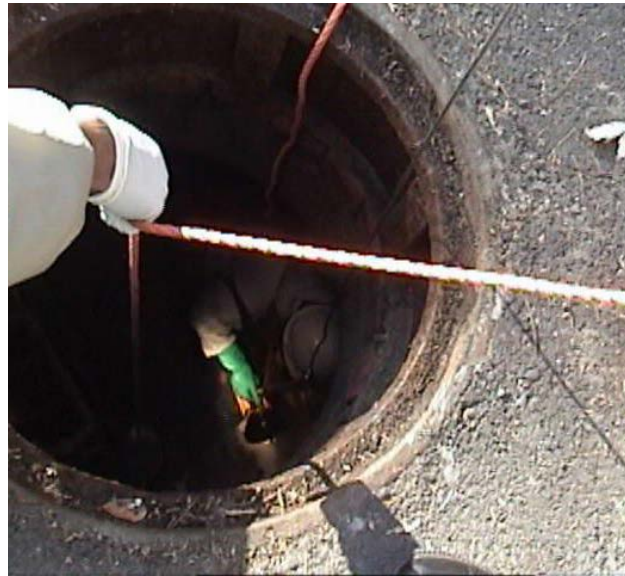
DEP staff begins sewer investigation
