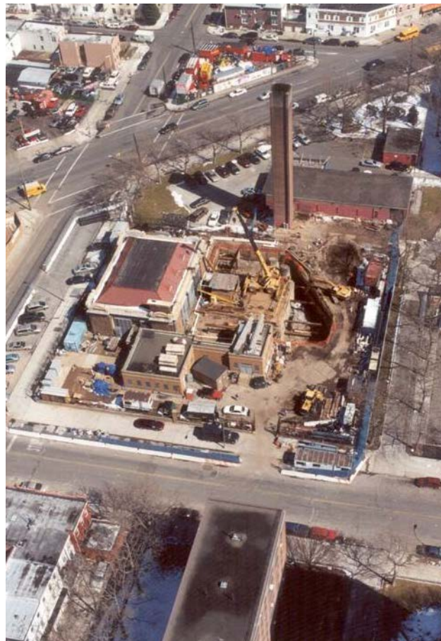
Construction at Avenue V pump station
