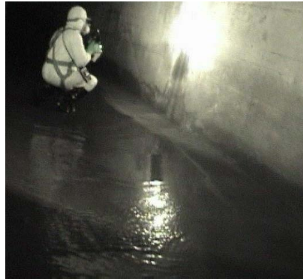
DEP staff conducts in-sewer investigation
