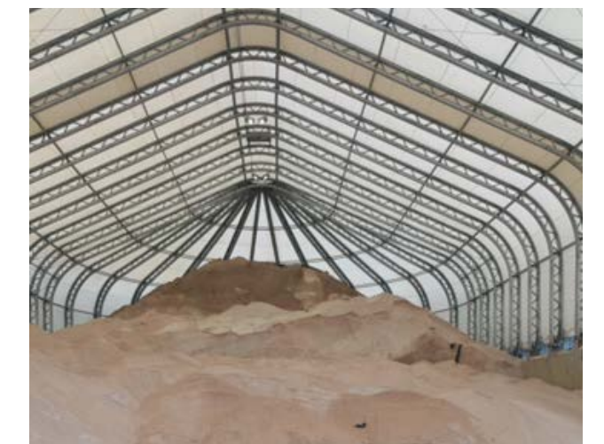
DSNY salt shed
