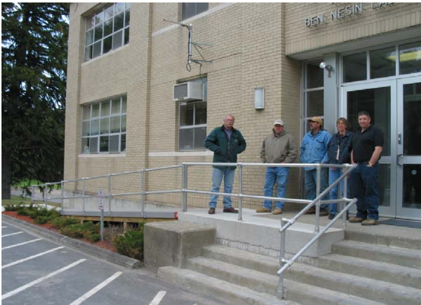
The new ramp at Ben Nesin Laboratory.
