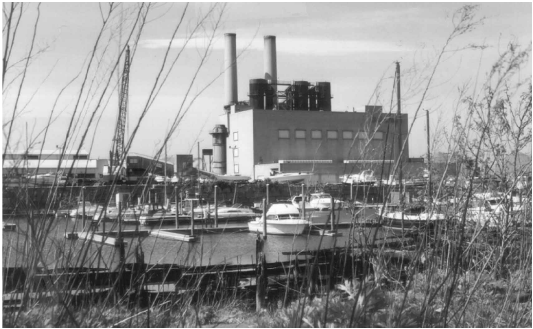
Figure 5.7-1: View northward from Bay 43rd Street. (Photo 2000)
