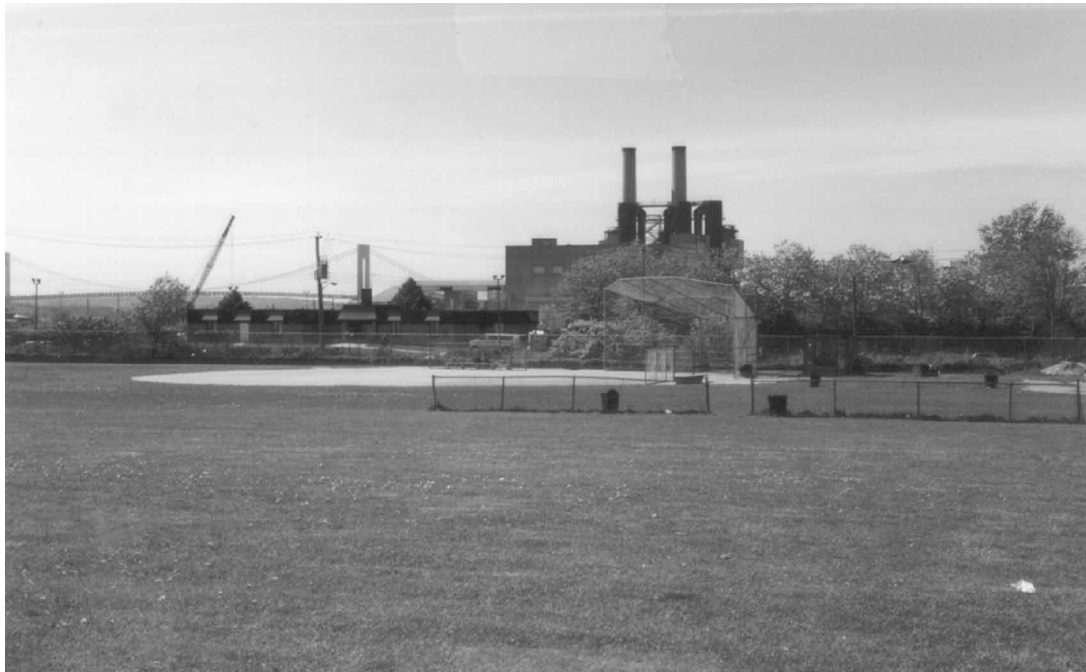
Figure 5.7-4 : View northward from the interior of Dreier-Offerman Park. (Photo 2000)
