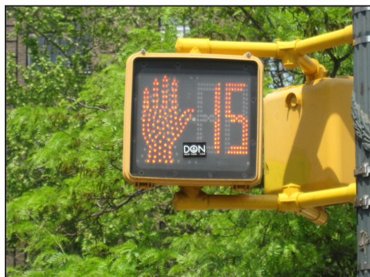
Countdown signals installed
