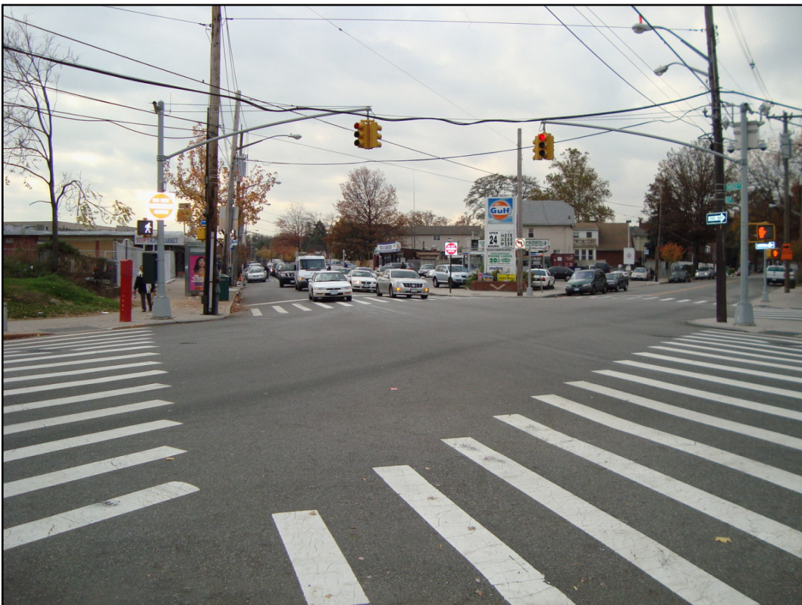
New conflict-free crossing with LPI installation
