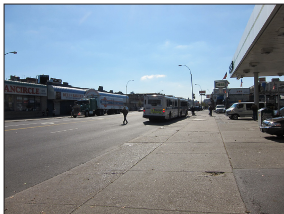
Existing mid-block bus stop encourages unsafe pedestrian crossings
