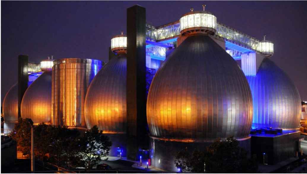
NYC Department of Environmental Protection Newtown Creek Wastewater Treatment Plant
