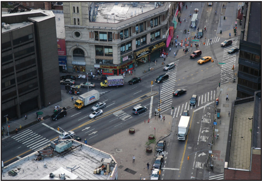
Before: Heavily skewed intersection of Flatbush Avenue and Nevins Street
