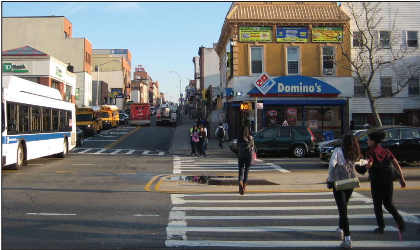
After: Improved crossings across 4th Avenue
