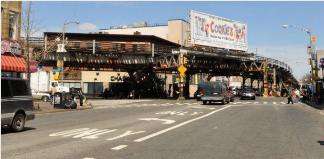
After: 4 to 3 conversion and left turn bay implemented
