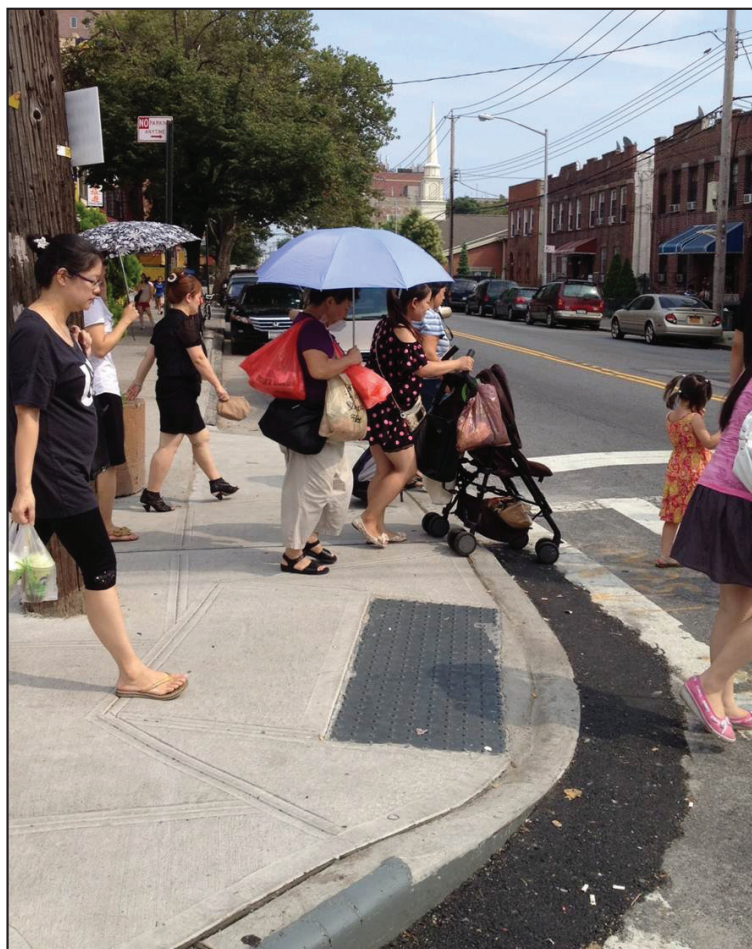
After: Curb extension shortens crossing distances for pedestrians and slows turning vehicles
