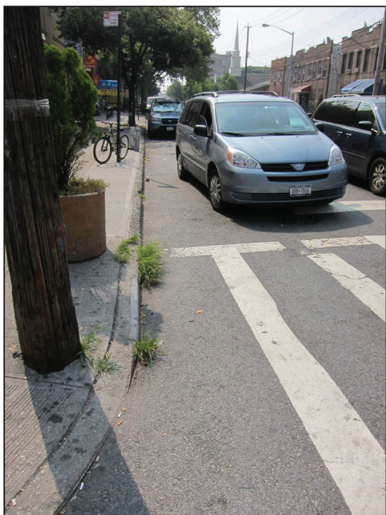
Before: High occurrence of pedestrian and vehicle conflicts
