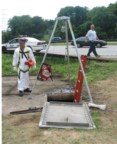
Confined Space Drill
