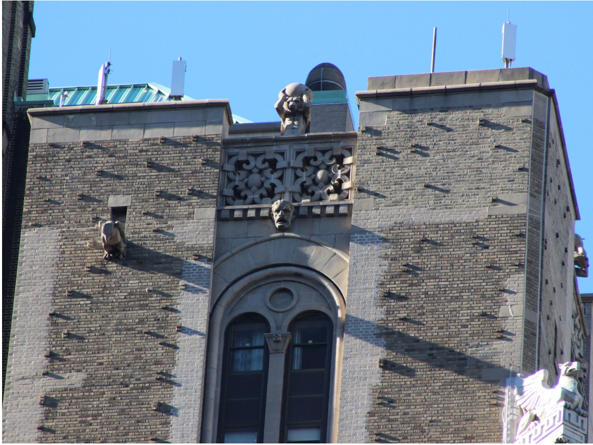
Decorative detailing upper stories east facade
