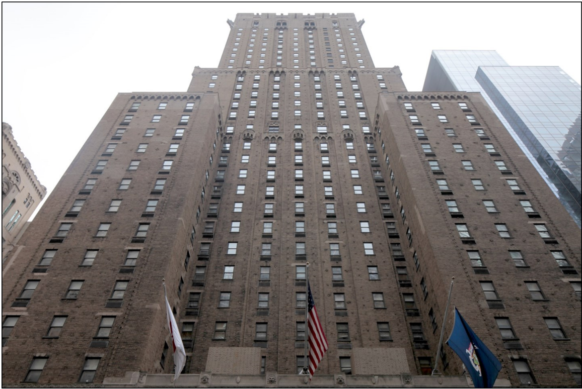
Upper stories Lexington Avenue showing battered wall treatment
