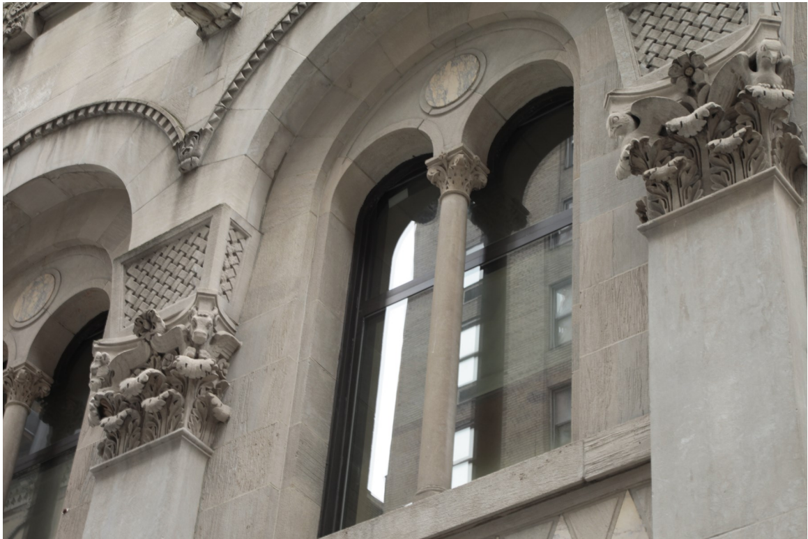
Detail, East 49th Street base Photo: Sarah Moses, June 2016
