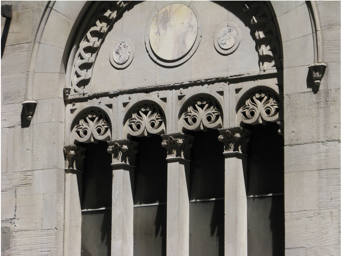
Detail, window surround East 48th Street base
