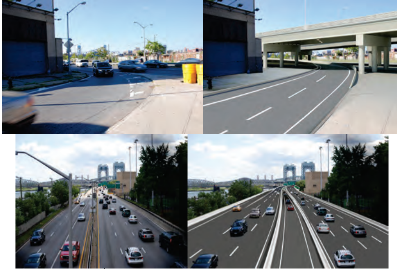
Looking East at 2 nd Avenue: Current and Proposed View. Looking South From 3 rd Avenue Bridge: Current Harlem River Drive and 2 nd Avenue Exit and Proposed Harlem River Drive With Left Lane Exit to 2 nd Avenue.
