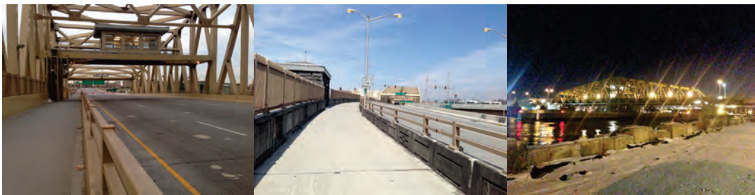
Willis Avenue Bridge in 2014.
