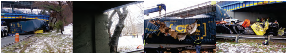
Damaged Bridge, Cargo Container, and Contractor Truck After An Over-Height Trailer Struck the Bridge in January 2012.
