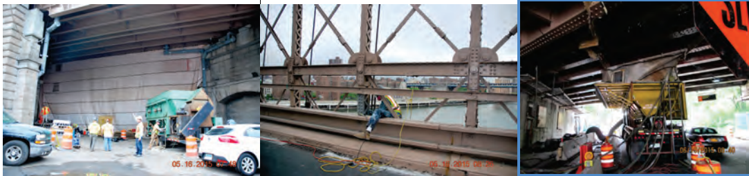
May 2015: Class 1A Abrasive Blast Containment System for the Main Street Structure Promenade Steel. Power-Tool Cleaning on Steel Repairs at the Suspended Spans. June 2015: Brooklyn Approach Structures.
