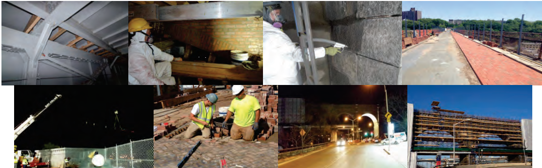
Winter 2014: Steel Stringer Installation. Spring 2014: Brick Repairs and Stone Cleaning. Summer 2014: Brick Installation. ADA Ramp Steel Installation. Summer 2014: Brick Installation. Winter 2015: LED Lighting on the Arch. Scaffolding. (Credit: NYCDDC)
