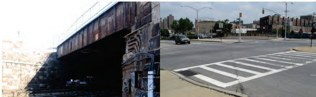
East 165 th Street Bridge over MNRR.
