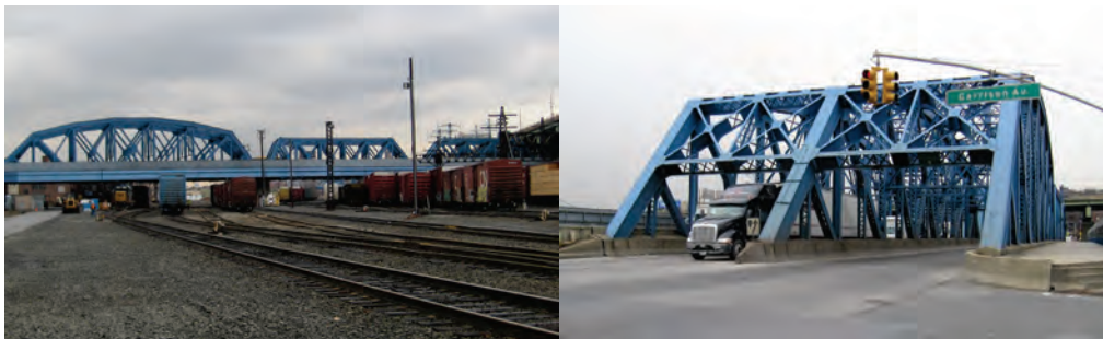
Leggett Avenue Bridge over Amtrak.
