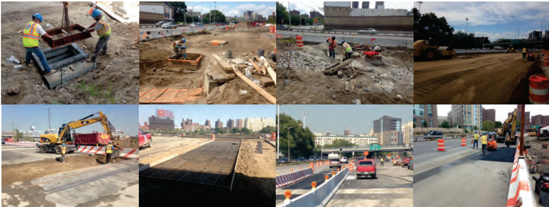
August 2015: Backfilling Utilities at Second Avenue. Contractor Working on the Temporary Roadway Placing the Sub-Base Second Layer. September 2015: Preparing New Concrete Crane Pads With Reinforcement. Painted Concrete Barriers Near Ramp C and Temporary Roadway. October 2015: Adjusting the Grading on the New Temporary Roadway. (Credit: Artemio Angeles)
