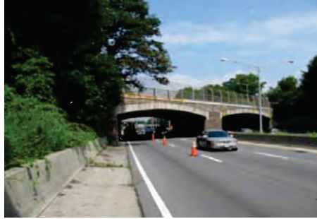
Douglaston Parkway Bridge Northbound Over Cross Island Parkway.
