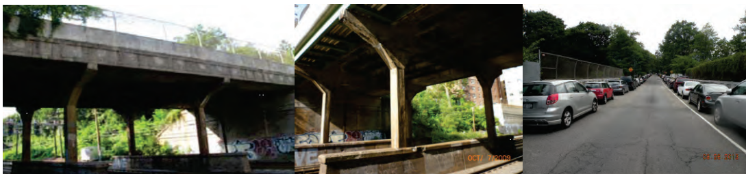
80 th Road Bridge over LIRR Main Line. Piers 1 and 2. End Approach. (Pier and Approach Credit: NYSDOT)
