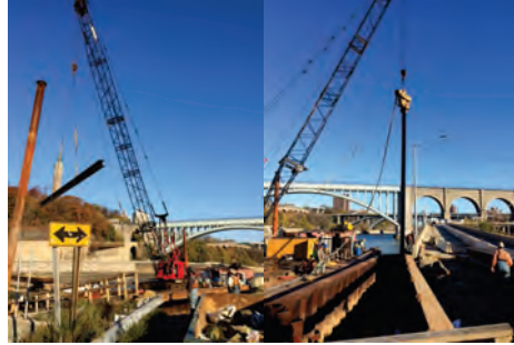
November 2015 - Depot Place over Conrail – Placing Piles to Build a Seawall.
