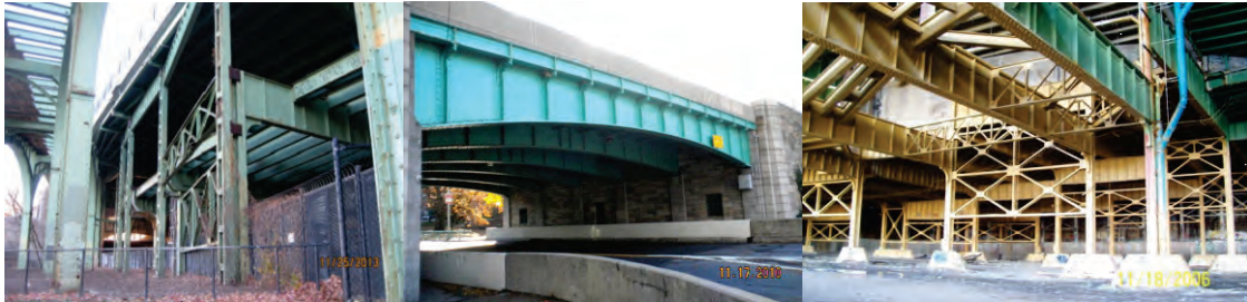
West 72 nd Street Viaduct Left Elevation Spans #1 -5, and Span #107. Piers #3 – 10. (Credit: NYSDOT)
