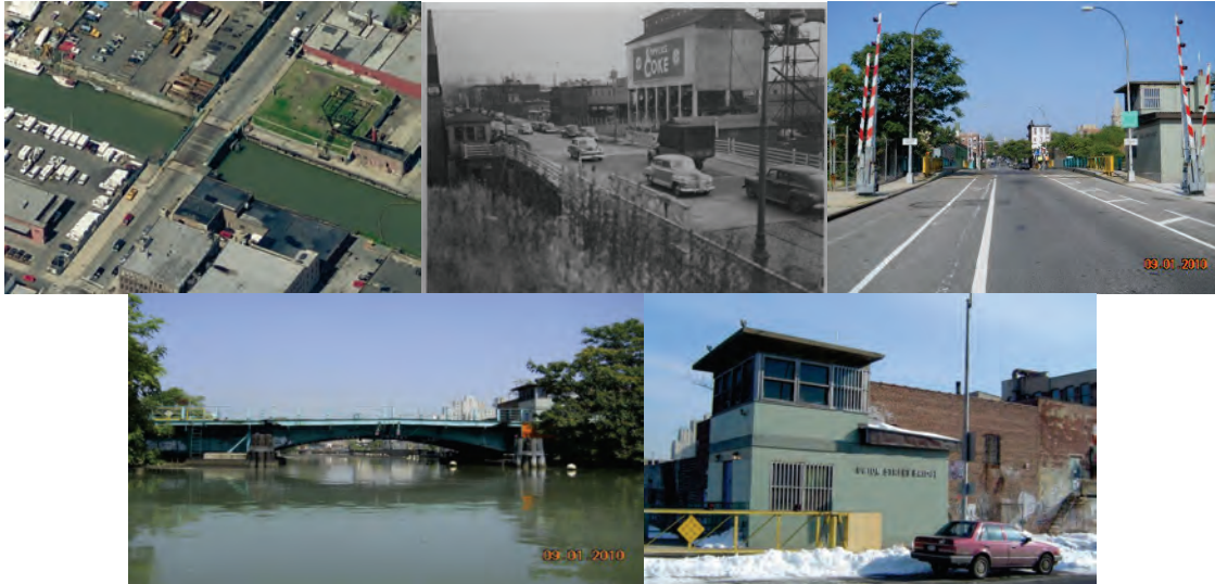
Aerial View of Union Street Bridge. Bridge in 1949 and 2010. (2010 Credit: NYSDOT) Operator House.
