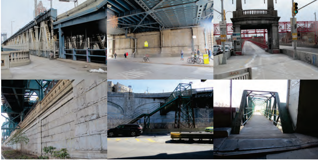
Winter Monitoring Locations: Manhattan, Williamsburg, Ed Koch – Queensboro Bridge, and West 155 th Street Pedestrian Bridge.
