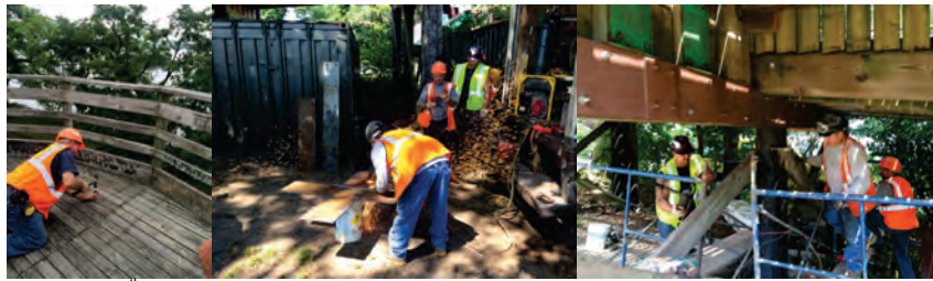
28 th Avenue Pedestrian Bridge over Cross Island Parkway in July 2015.
