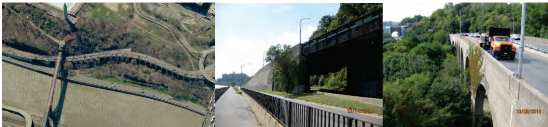
Aerial View. Trans-Manhattan Expressway Connector Ramp in 2014: Elevation Right Spans 1 – 25, 33 – 40. (Credit: NYSDOT)
