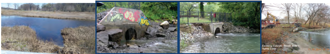
Turtle Cove. Existing Culvert – South Side.
