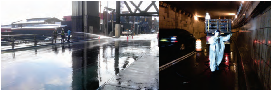
Water Spraying the 9 th Street Bridge over Gowanus Canal in July 2012. July 2013: Power Washing the Battery Park Underpass. (Credit: Earlene Powell)
