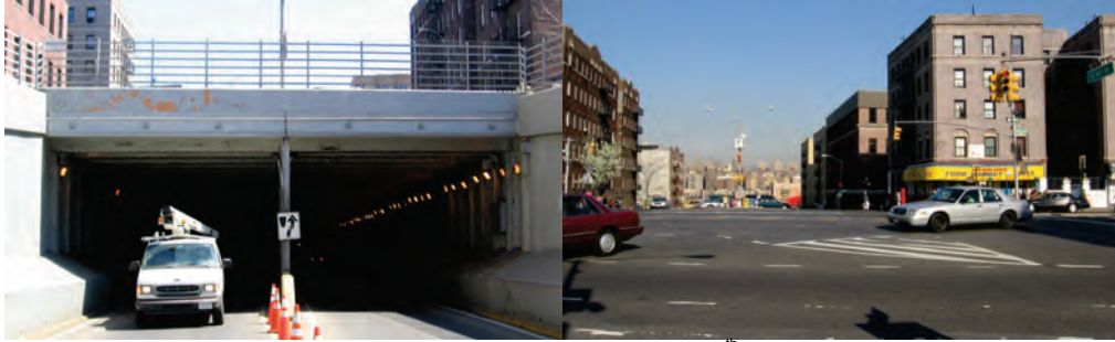
Grand Concourse Bridge over East 167 th Street.
