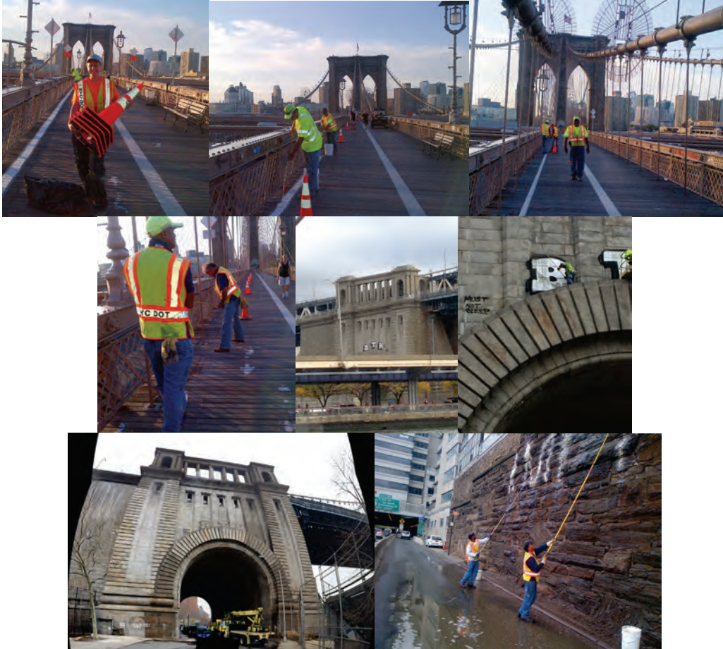
August 2015: Brooklyn Bridge Line Striping. Bridge Painter Elisangela Oliveira. Bridge Painters Arlindo Lima and Carlos Mata. Bridge Painter Willie Tyler Checking the Striping. Bridge Painter Gerson Do Rosario and Supervisor Bridge Painter Cesar Pazmino. (Credit: Earlene Powell) March 2015: Supervisor Bridge Painter Goncalo Lima Removing Graffiti on the Manhattan Bridge Arch on Cherry Street. (Credit: Cesar Pazmino) July 2015: Bridge Painters Gerson Do Rosario and Carlos Mata Removing Graffiti on the FDR Drive.
