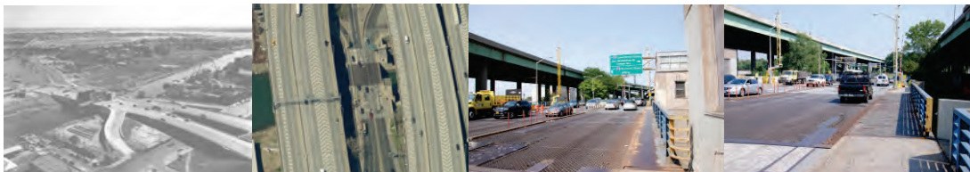
Unionport Bridge in 1953 and 2009. Existing Bridge North Sidewalk and Movable Span Looking West. Looking east at the south sidewalk.
