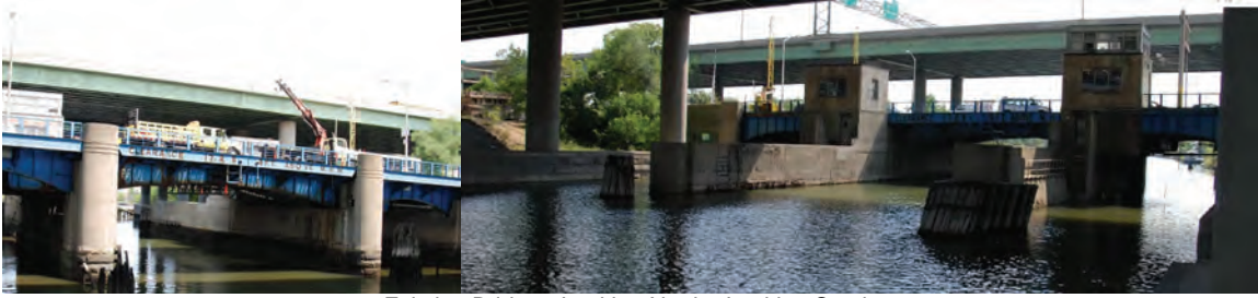
Existing Bridge - Looking North. Looking South.
