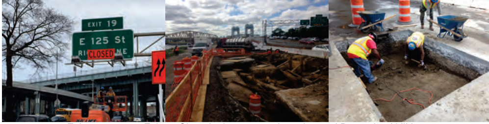
February 2015: Exit 19 Closed. June 2015: Locating and Removing Utilities.
