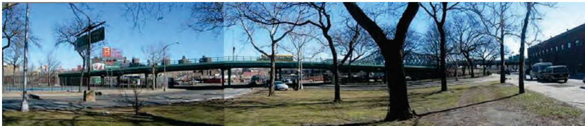
Harlem River Drive Bridge at East 127 th Street.
