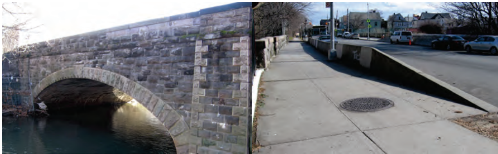
East 180 th Street Bridge over Bronx River.
