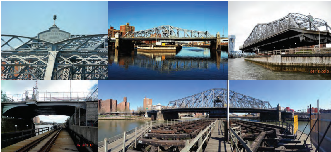
Madison Avenue Bridge Sign in 2007. (Credit: Duane Bailey-Castro) Bridge in 2009. (Credit: Bernard Ente) General View of Truss Swinging in 2010 and Right Elevation of Span 15 in 2012. (Credit: NYSDOT) North Elevation View.
