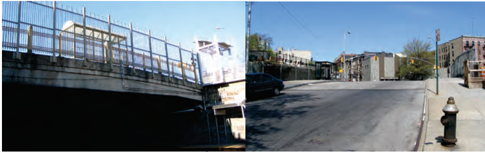
East 162 nd Street Bridge over MNRR.
