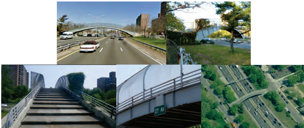
27 th Avenue Bridge – Existing Conditions.
