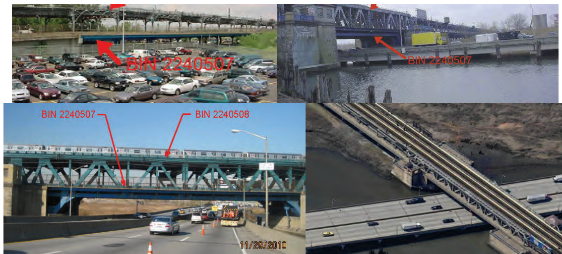
Roosevelt Avenue Bridge (#2240507) in 2002, 2004, and 2010. (Credit: NYSDOT) Aerial View.
