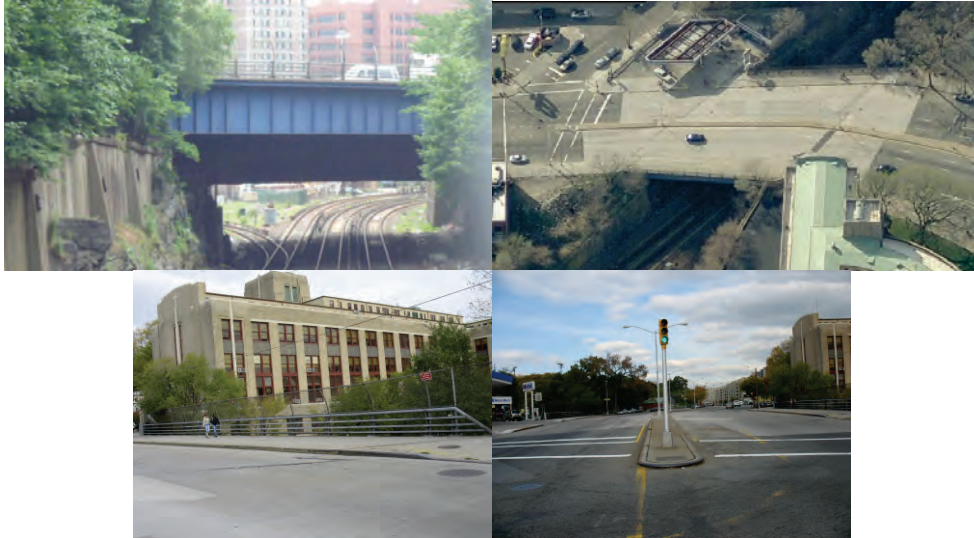
Grand Concourse Bridge over Metro North in 2010. (Credit: NYSDOT) Aerial View. Sidewalk and Top of Bridge.
