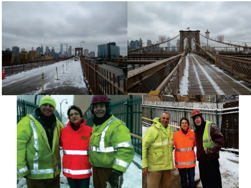
Snow Removal on the Brooklyn Bridge in January 2015. (Credit: Russell Holcomb) Commissioner Polly Trottenberg Visiting Division Staff After the January 2015 Snowstorms: Carpenters Edward Alfano Jr. and Gregory Nolan, Supervisor Carpenter Joseph Vaccaro and Cement Mason Stephen Buckley.
