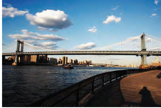
Manhattan Bridge in 2014. (Credit: NYSDOT)
