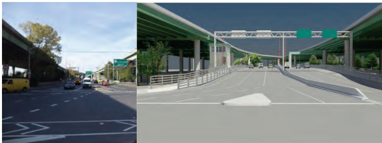
Looking West – Towards Current And Proposed Bridge.
