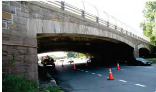
Douglaston Parkway Bridge Southbound Over Cross Island Parkway.
