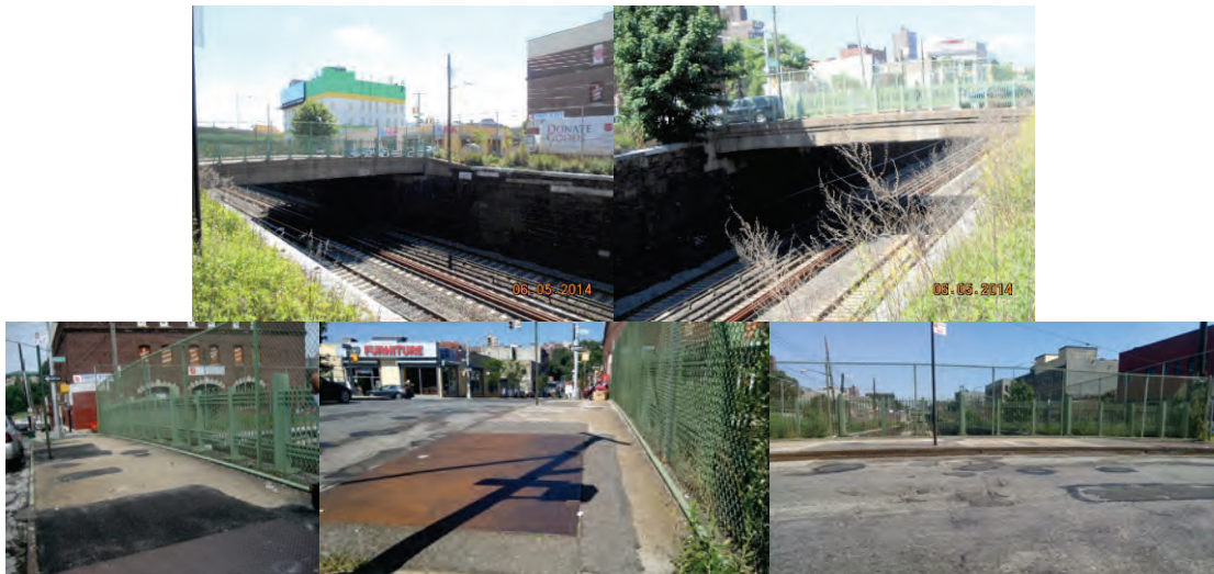
2014: East 175 th Street Bridge Left and Elevations. (Credit: NYSDOT) Sidewalk conditions.
