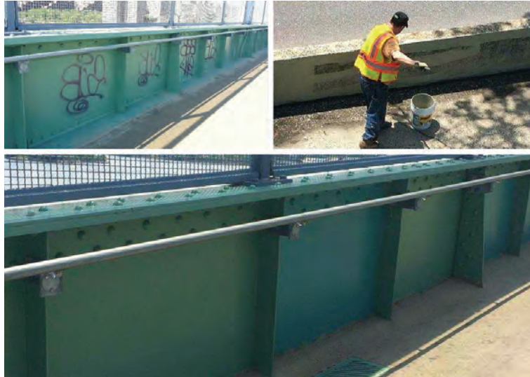
Removing Graffiti from Wards Island in June 2015.
