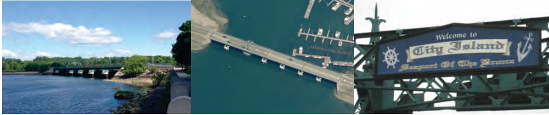
View of City Island Bridge From the Esplanade. Aerial View of Current Bridge. Welcome Sign.
