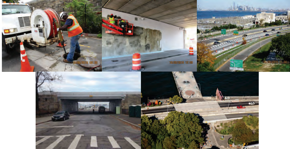
October 2015: Post-Construction Drainage Cleaning and Inspection at Southwest Abutment. Applying Protective Sealant to the East Abutment Wall. Belt Parkway Roadway at West Side of Bridge. NYCDEP Owl's Head Waste Water Treatment Plant at Top. November 2015: Construction Complete.
