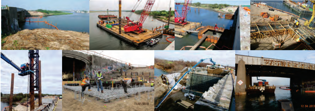
June 2013: North Side of Gerritsen Bridge - Turbidity Curtains Placed on Both Sides of Navigable Channel. July 2013: Work Barges Driving Steel Sheeting for Pier #1 Cofferdam. September 2013. October 2013: Rebars and Form Work for Footing and Walls at the Northwest Abutment. Stage 1 Piles. November 2013: Inspecting Rebar. December 2013: Tremie Concrete Pour at Pier #2. Inspecting Spans 7 & 8 of the Existing Bridge From a Barge. (Inspection Credit: NYSDOT)
