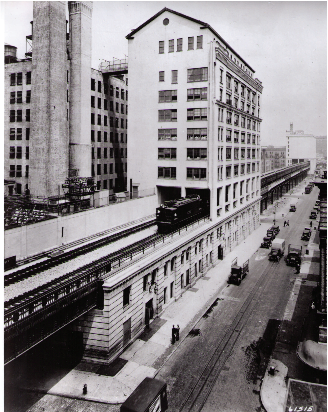
Bell Telephone Laboratories Complex (including former Western Electric Company Building) (now Westbeth Artists' Housing) , showing Sections G and H after construction of the New York Central Railroad elevated freight railway (1934)
