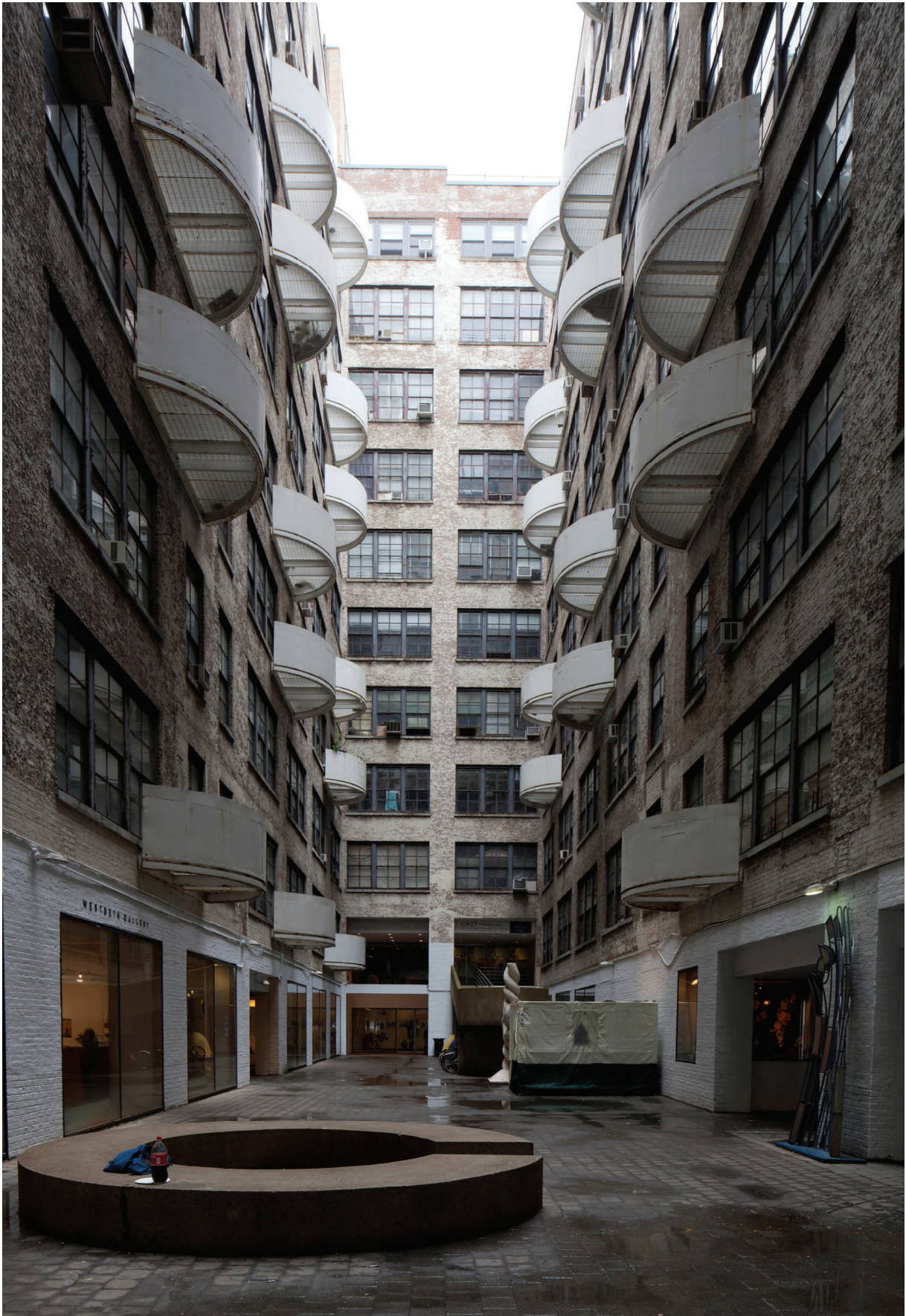
Bell Telephone Laboratories Complex (former Western Electric Company Building) (now Westbeth Artists' Housing), Sections A-D, Interior Light Court
