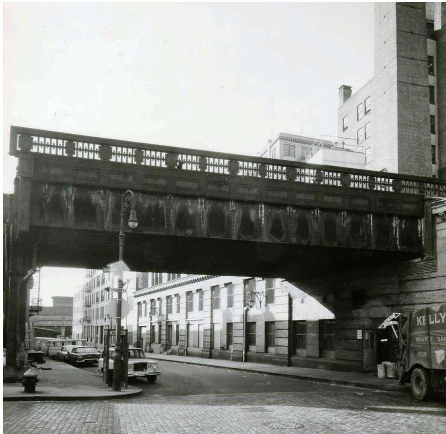
Bell Telephone Laboratories Complex (former Western Electric Company Building), Section G
