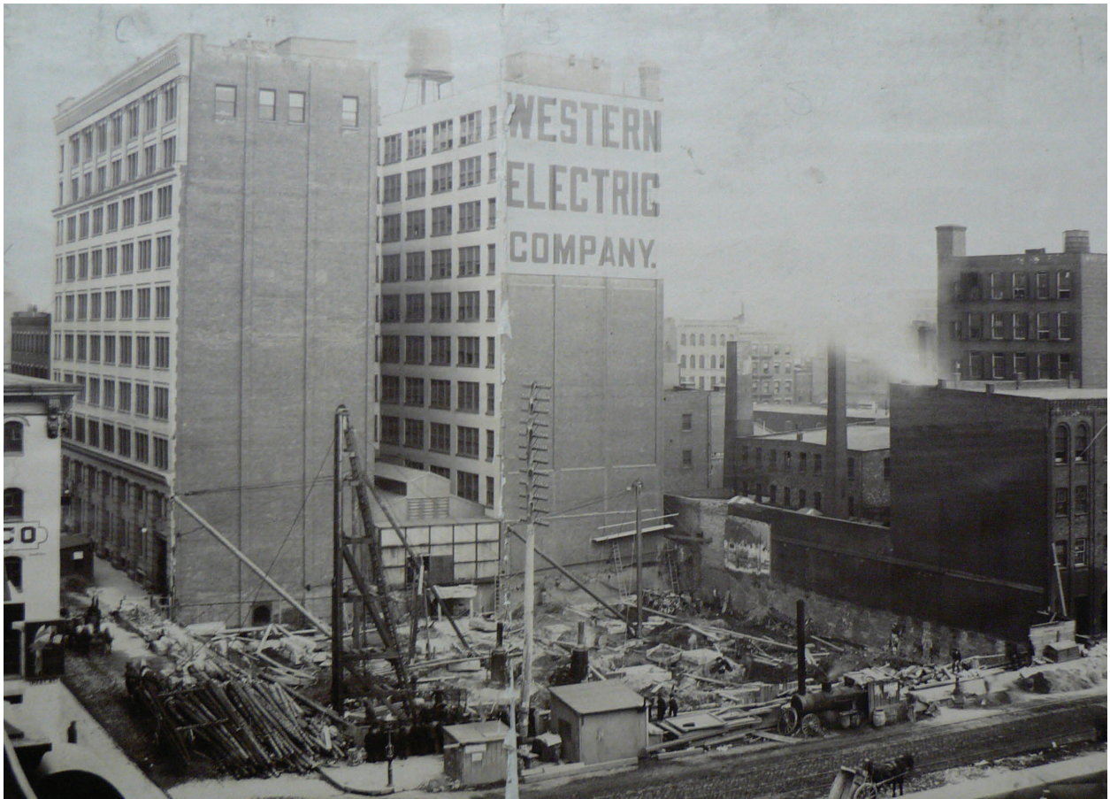
Western Electric Company Building, Sections C and B, and Hook's Steam-powered Factory Building (Section I)
