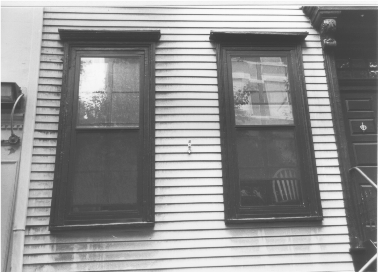
Detail of First Floor Windows
