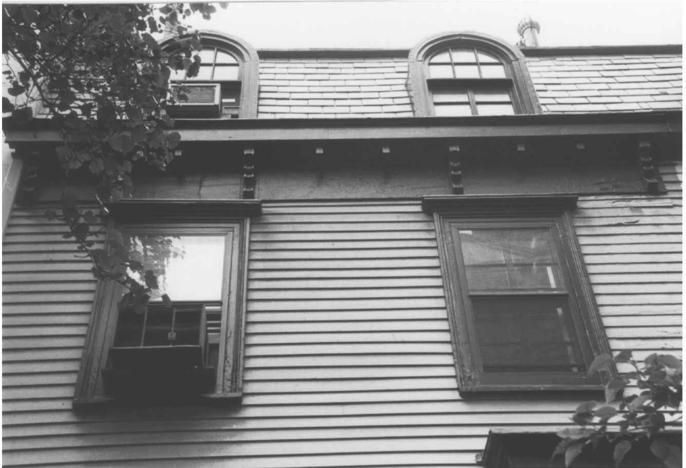
Detail of Second Floor Windows and Mansard Roof
