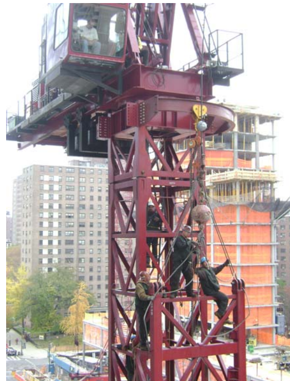
Figure C.8.4: Dismantling process
