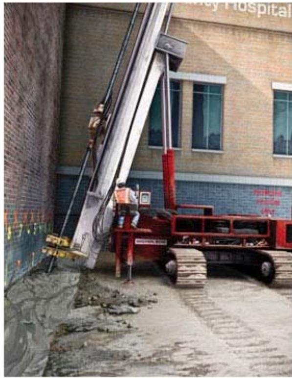
Figure D.16.10: Jet grout underpinning (Nicholson Construction Company)
