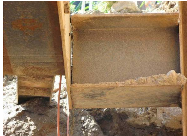
Figure D.14.3: Typical braced retention system. Close-up at right of inadequate (omitted in this case) weld at stub connection to waler.
