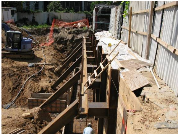
Figure D.14.3: Typical braced retention system. Close-up at right of inadequate (omitted in this case) weld at stub connection to waler.
