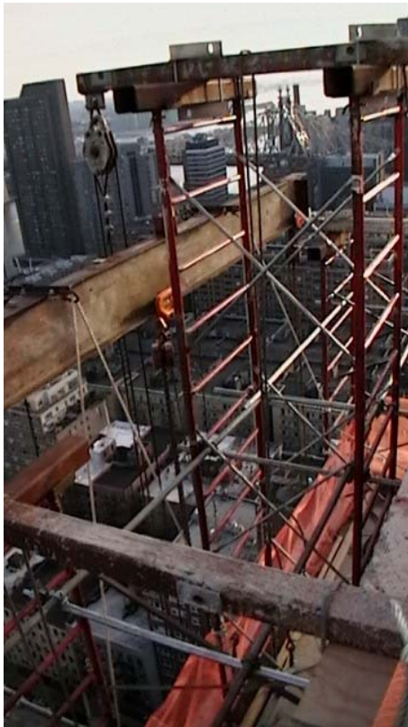
Figure C.8.16: Scaffold structure for hoist (Site C-52, 12/18/08)
