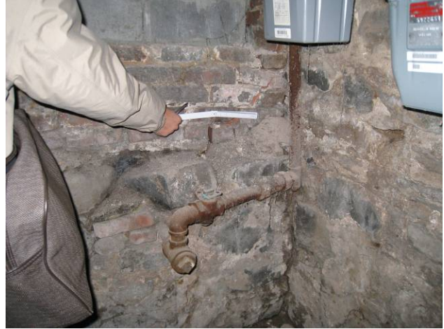
Figure D.10.4: Cracking and lateral displacement of below grade wall during underpinning
