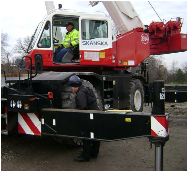
Figure C.9.11: DOB Inspecting a Mobile Crane
