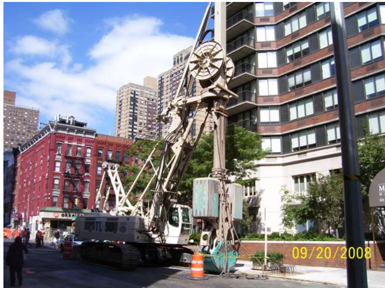
Figure D.16.5: Slurry wall rig with hydraulic grab
