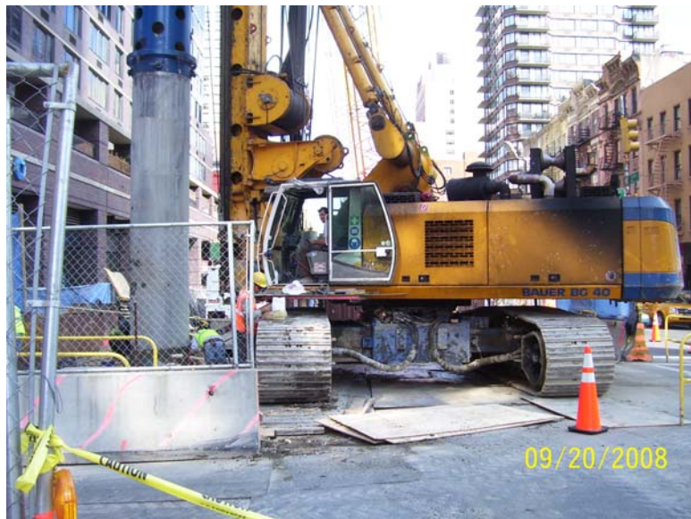
Figure D.16.4: Secant piles being installed using segmental casing
