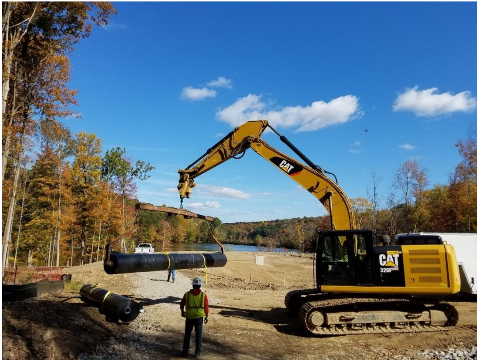
Figure 4.20 Drewville Road stormwater basin during installation of liner
