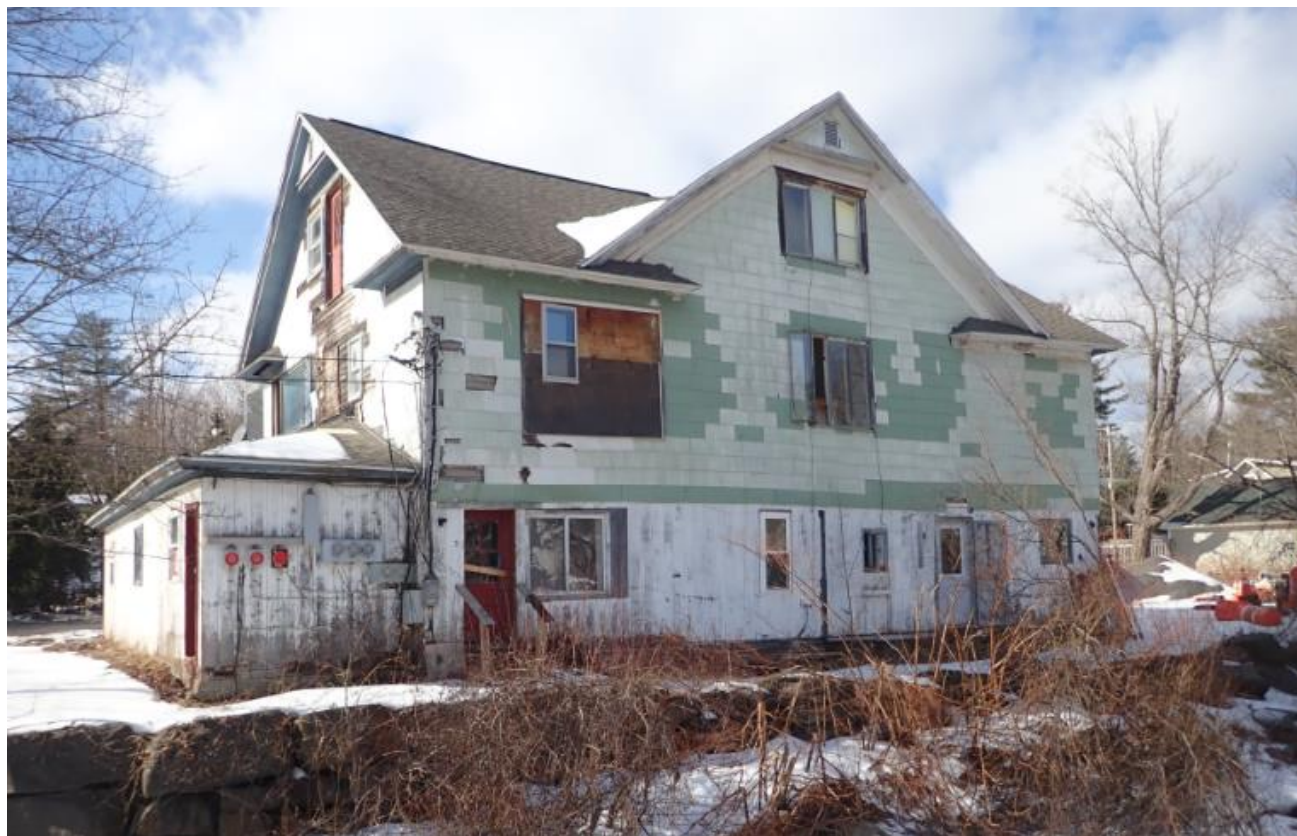
Figure 4.3 This 0.4-acre property with its flood-prone building in the Village of Tannersville, Greene County was signed to purchase contract in 2019 and will be acquired under the NYC-Funded Flood Buyout Program. NYC will pay for the acquisition but the village will own and manage the land.
