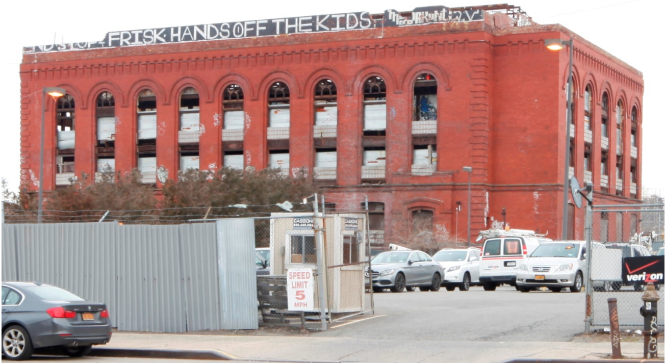
BRT Engine House, south and east facades Sarah Moses, LPC, 2017
