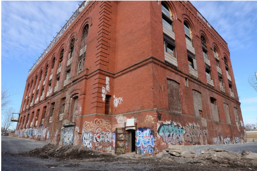
BRT Engine House South and east facades Powerhouse Arts, November 2013
