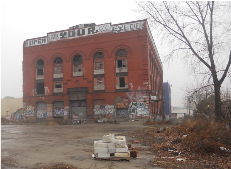
BRT Engine House, west facade Powerhouse Arts, 2014
