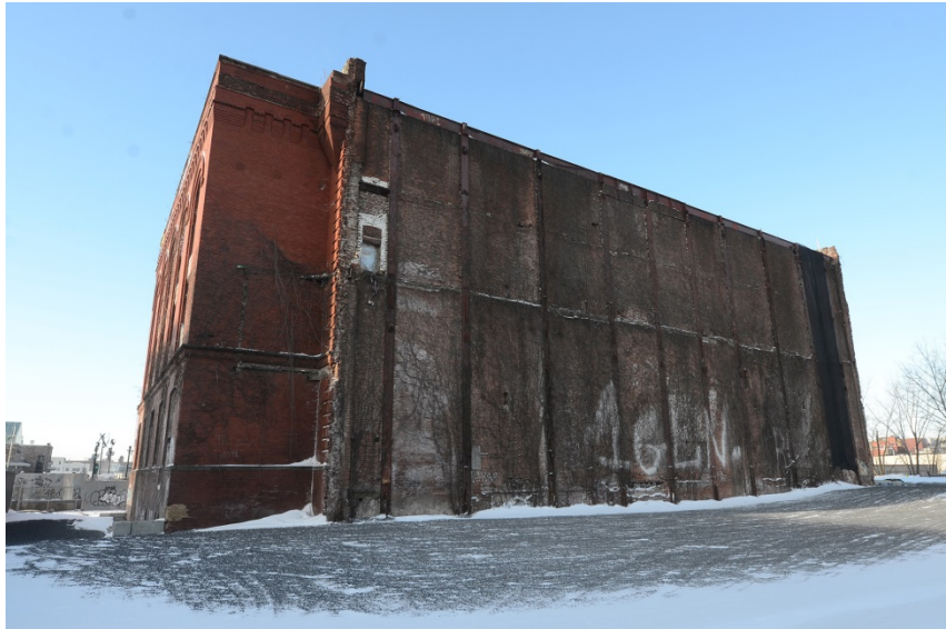
BRT Engine House North facade Powerhouse Arts, 2014
