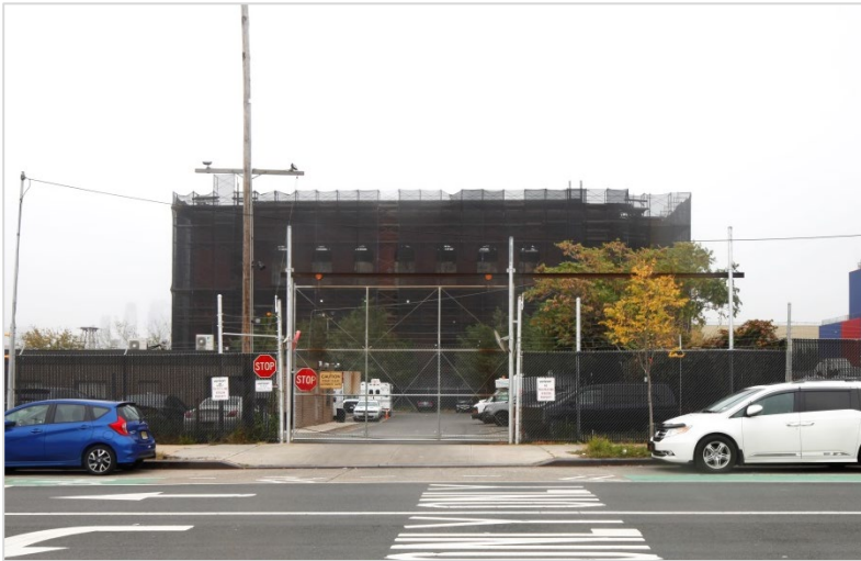
BRT Engine House View from 3rd Street LPC, October 2019
