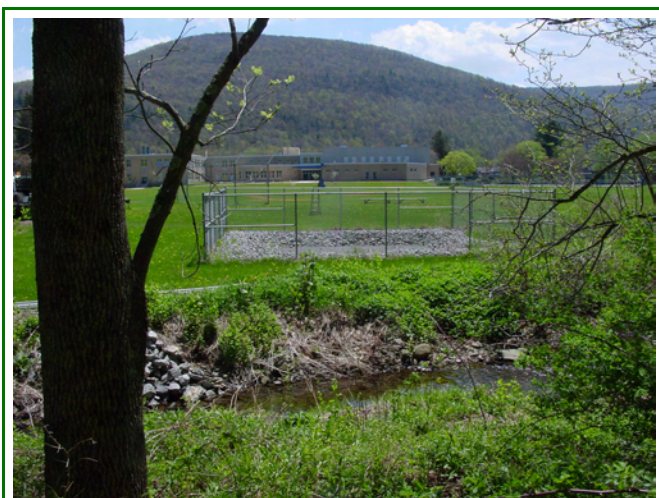
Figure 4.6 Sand filter portion of a stormwater retrofit installed at the Margaretville Central School bus garage, Pepacton Reservoir watershed.
