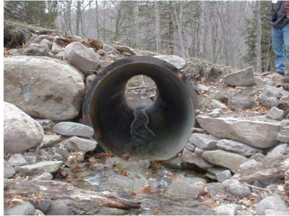
Figure 4.7 A properly installed timber harvest road culvert, a project of the Forestry Management Program, Neversink Reservoir watershed.
