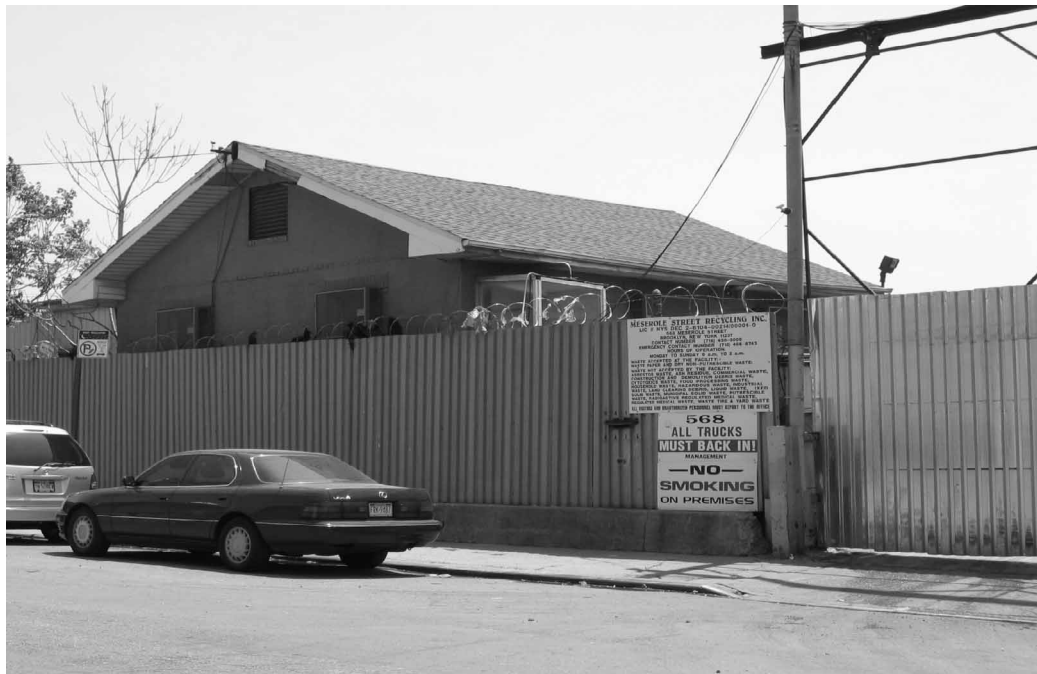
Figure 31.7-2 : Meserole Street Recycling Facility (Lot 2).
