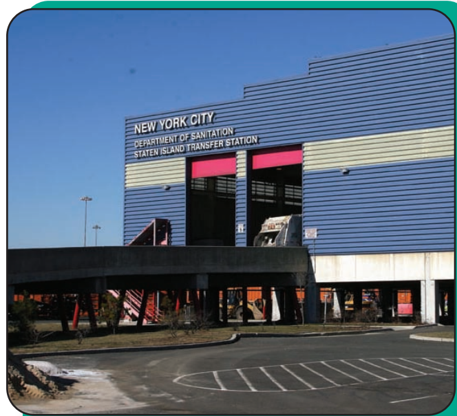
STATEN ISLAND TRANSFER STATION
