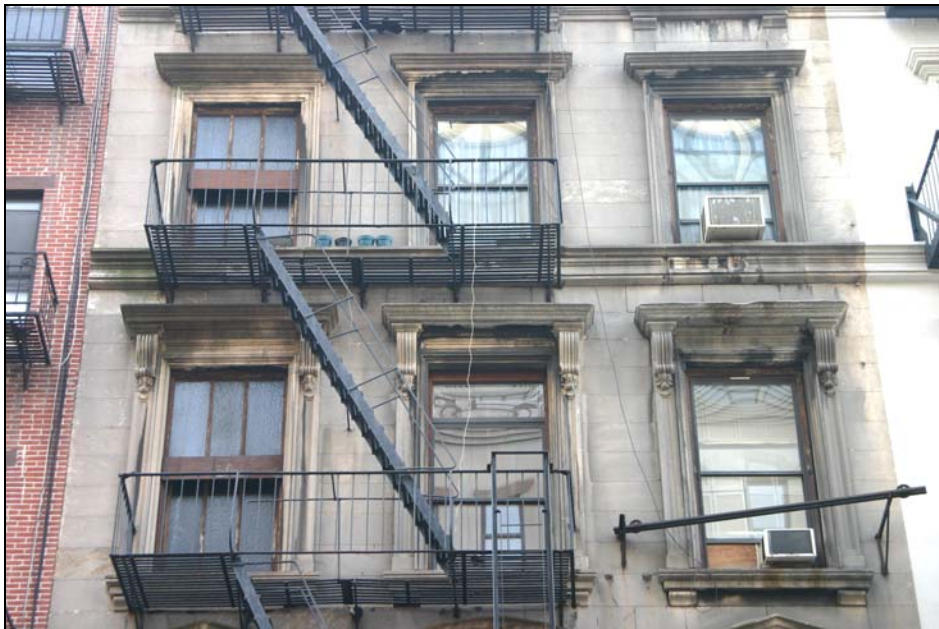
23 Park Place Building , 20 Murray Street elevation, details Photos: Carl Forster
