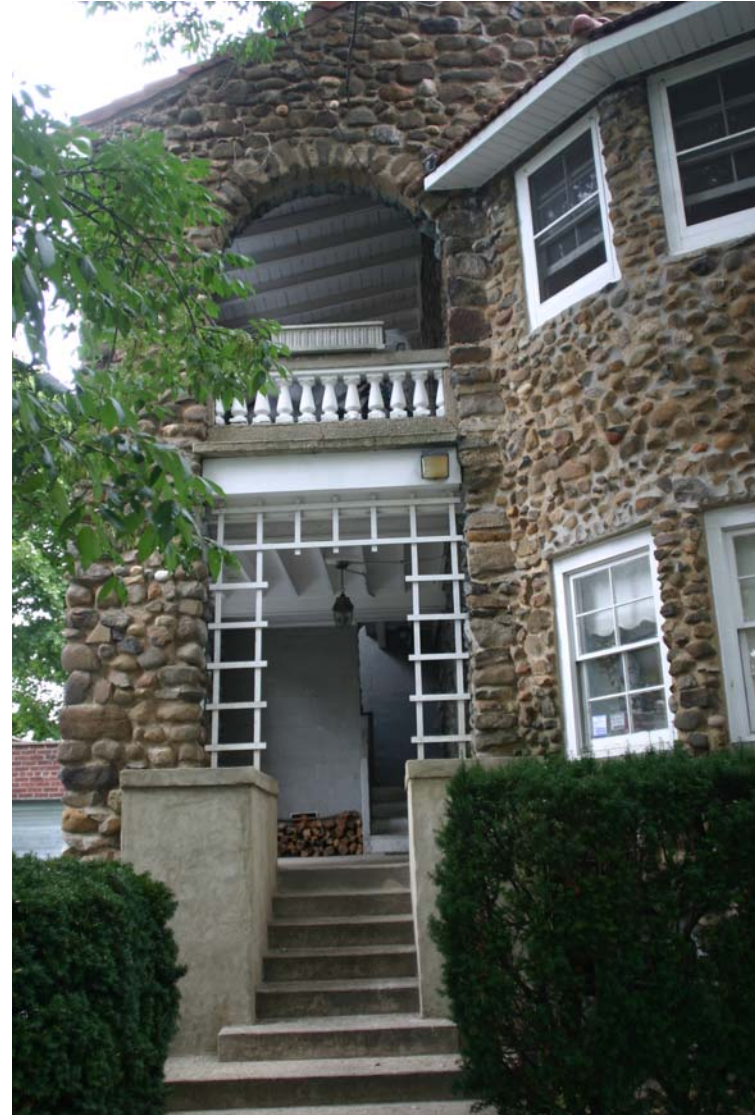
35-34 Bell Boulevard , rear entrance facing 36th Avenue Photo: Carl Forster
