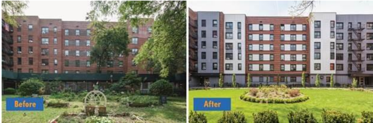
Before and after exterior renovations at 572 Warren Street. Photos provided by the Brooklyn Bundle PACT partner team.
