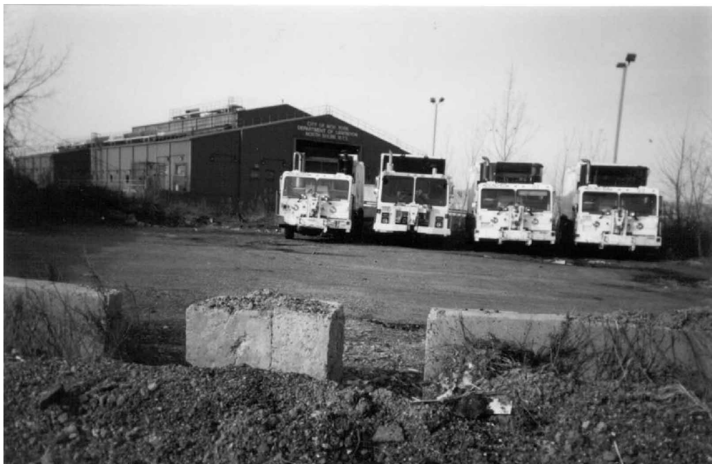
Figure 7.7-1 : View of MTS from 31st Avenue.
