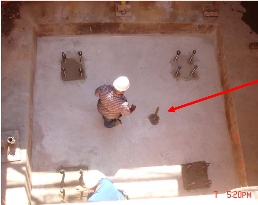
Figure C.7.9: Poured Foundation (Site C-78, 8/7/08)
