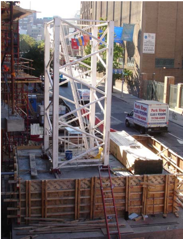
Figure C.7.8: Tower Crane Foundation (Site C-3, 9/5/08)
