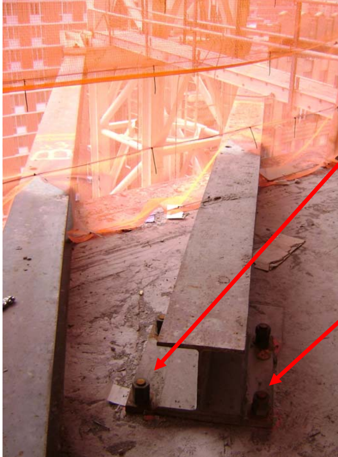
Figure C.7.4: Friction Connection Bolts (Site C-88 – 1/5/09)
