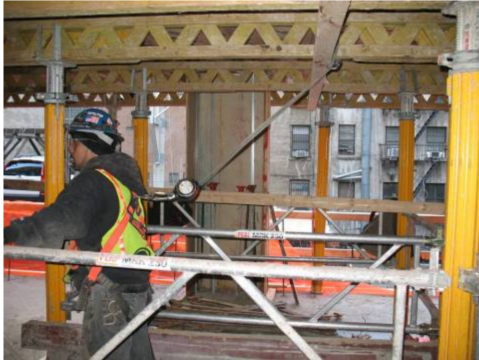
Figure B.8.4: Tie-off to Formwork Substructure Using Retractable Lanyard
