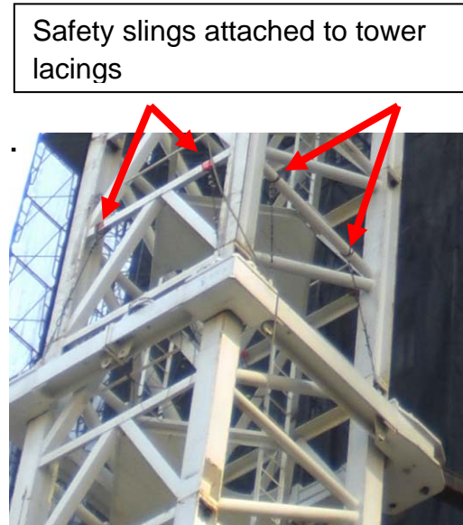
Figure C.7.5: Safety Slings at Site C-62.
