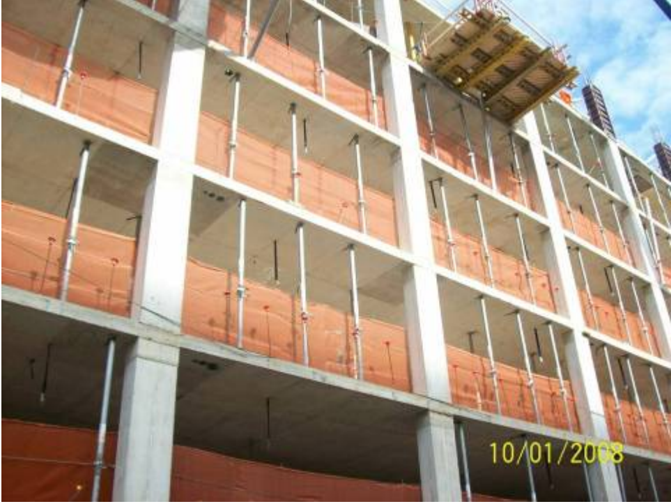
Figure B.7.17: Acceptable Outrigger System for Material Handling Near Active Floors (Top)
