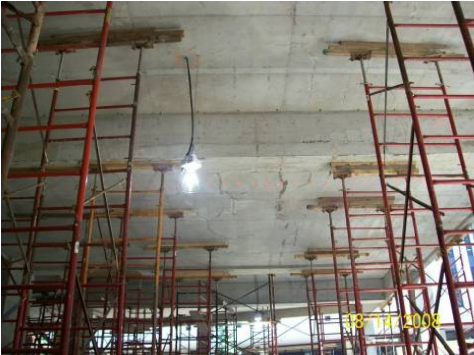
Figure B.6.3: Improved Filler Material Installation (Laid Horizontally) between Steel Shoring Tower and Concrete Soffit
