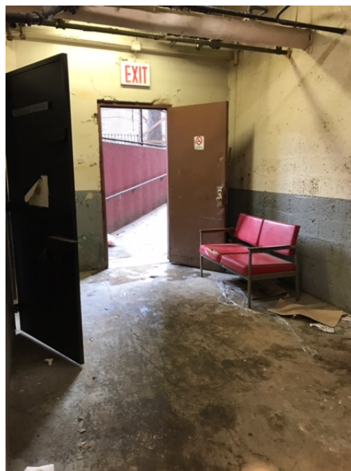
Photograph No 7 – Emergency Exit Door Does Not Open in the Outward Direction at Patterson Houses Senior Center
