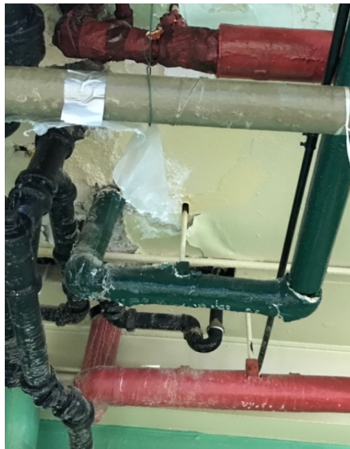
Photograph No 6 – Cracked Ceiling in Dining Room Area at Patterson Houses Senior Center
