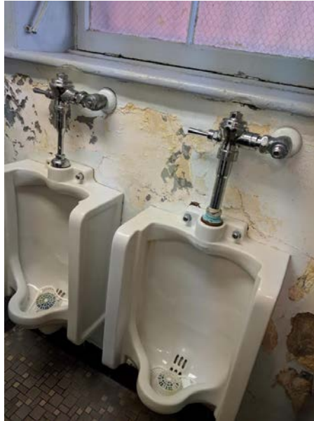
Photograph No 3 (a) – Peeling Paint on the Wall in Men’s Bathroom at Prospect Hill Neighborhood Senior Center
