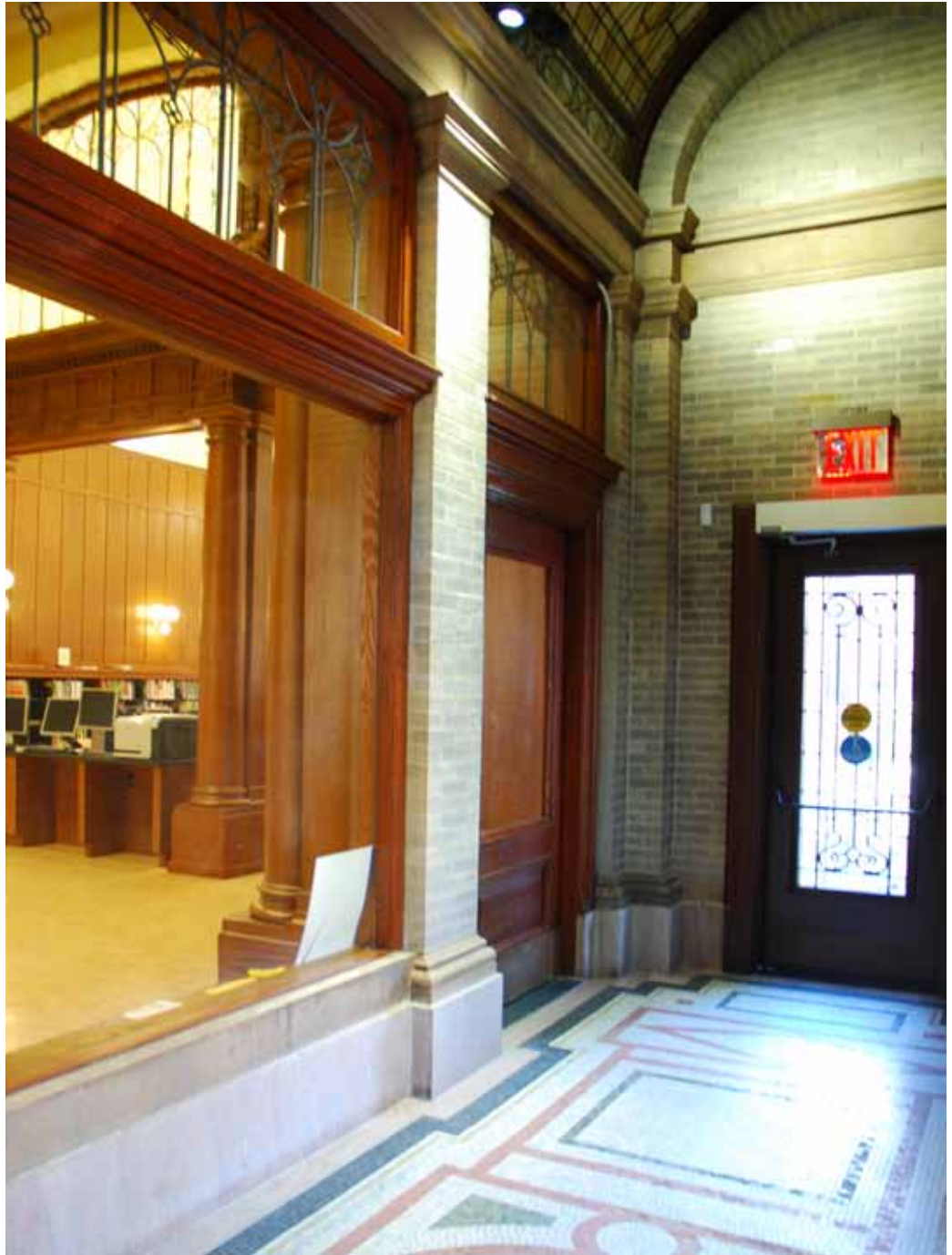
A-25. Vestibule looking south to new accessible door
