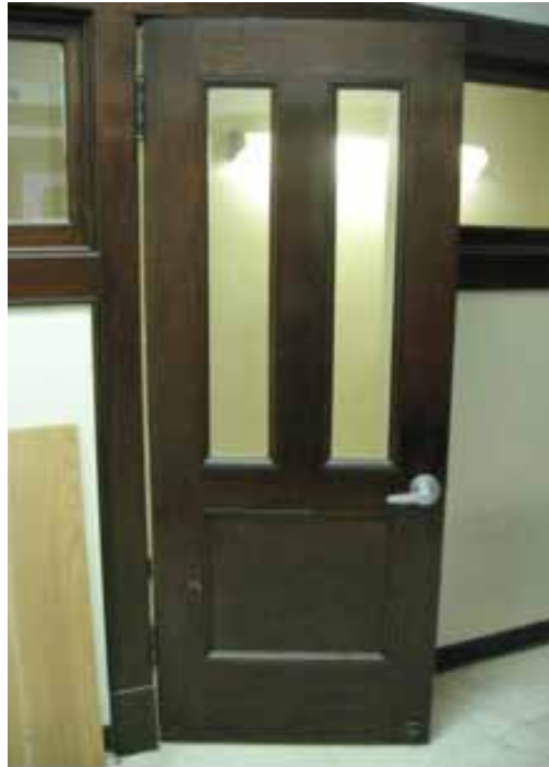
Figure 70. Another original oak door, flanked by transom windows. This view looks out from the reception room to the corridor.
