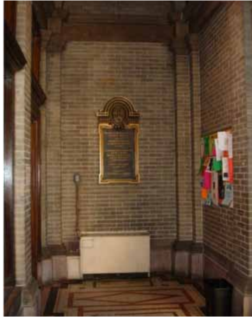
Figure 57. The main vestibule looking south towards the location of the new accessible door. The original plaque will be relocated to the opposite wall.
