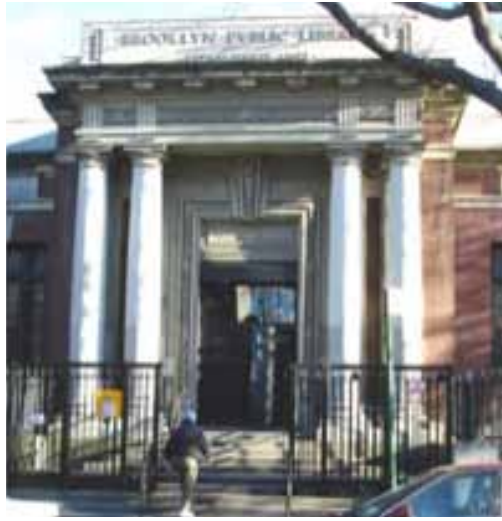
Figure 18. Main entrance showing the 1979 doors, transom, and light box and the newer picket fence extending across the stoop. Photo is ca. 2010.
