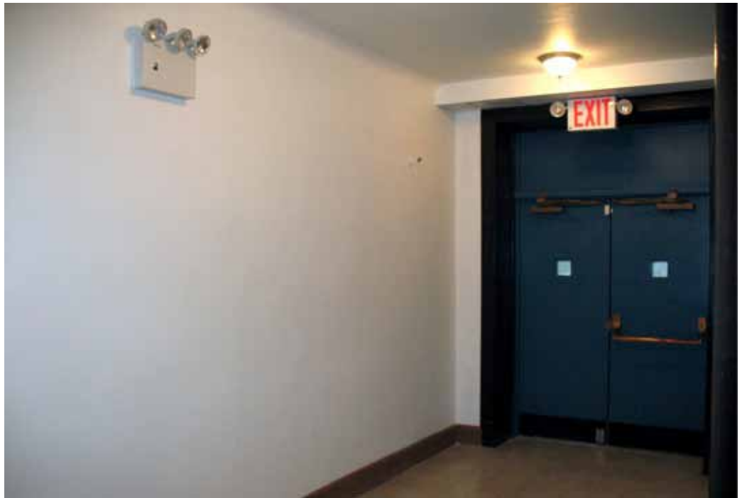
A-32. Lower vestibule looking north
