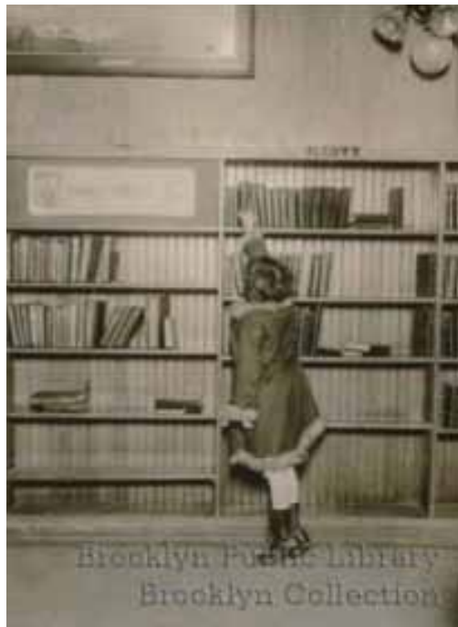
Figure 45. Original wood shelving in the Children's Room, showing the beadboard backing.
