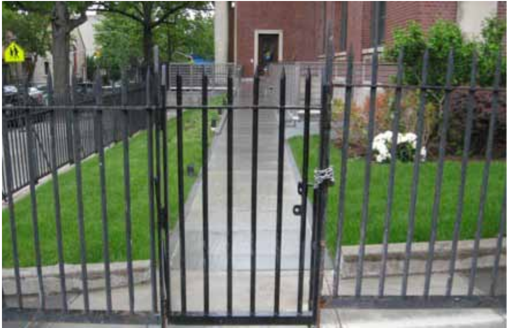
Figure 26. The phase 1 accessible entrance, including a new gate, bluestone walk and curbs, lights, bridge over the areaway, and new limestone-trimmed door into the Vestibule.
