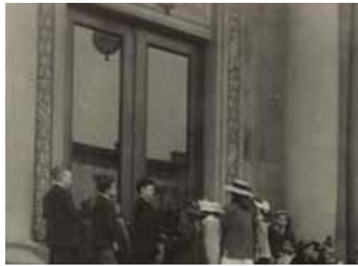
Figure 12. Original wood and glass entrance doors, without ironwork or transom.
