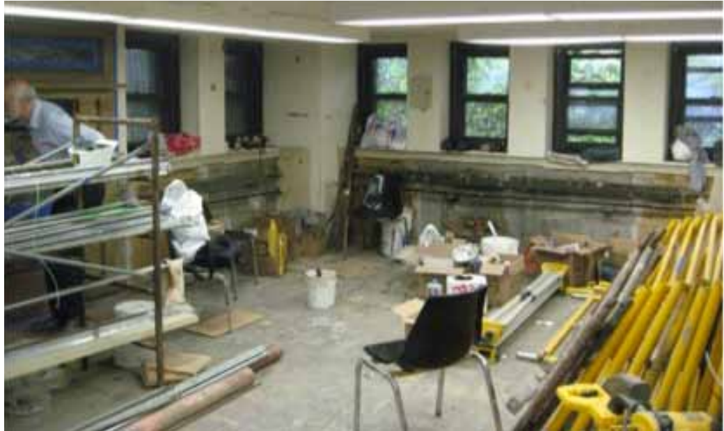
Figure 62. Original 1st floor reference alcove, now a staff workroom.
