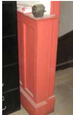
Figure 76. A bit of original "batten wainscot" is visible near the study room door. Extensive original woodwork remains in this room (see also fig. 66).
