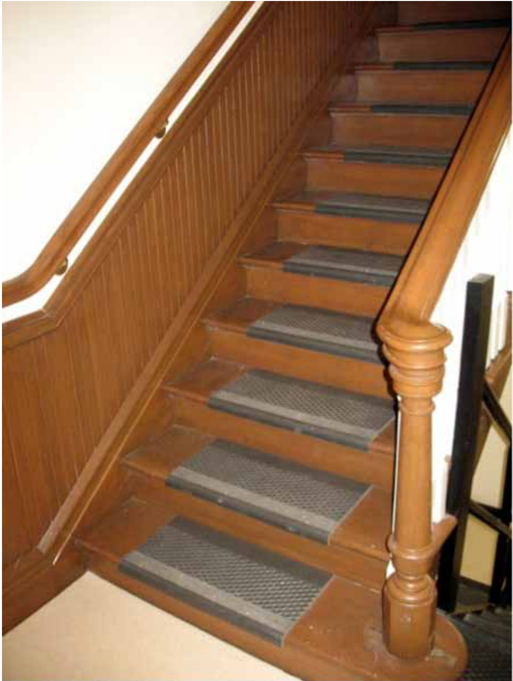
A-22. Staircase to mezzanine
