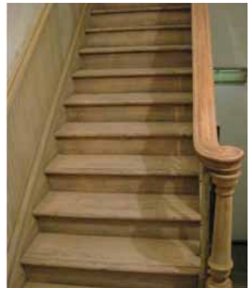
Figure 44. South staircase after stripping and before refinishing.
