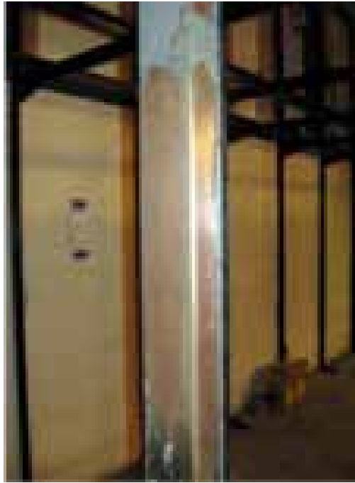
Figure 60. Test stripping of an end pilaster revealed the original bronze plating.
