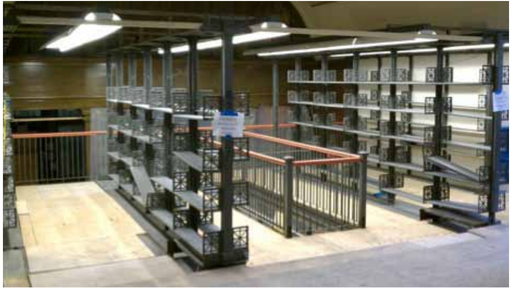
Figure 59. Pre-phase 3 construction showing second level of original Library Bureau stack system, including railings, vertical standards (originally bronze plated), shelves and bookend brackets (originally painted black). Glass floor remains under vinyl tile and plywood. Lights probably date from the 1950s.
