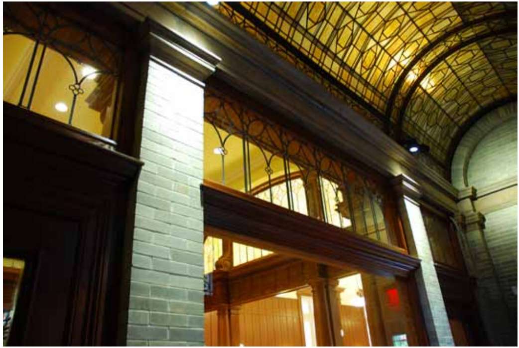
A-26. Vestibule lay light and transom
