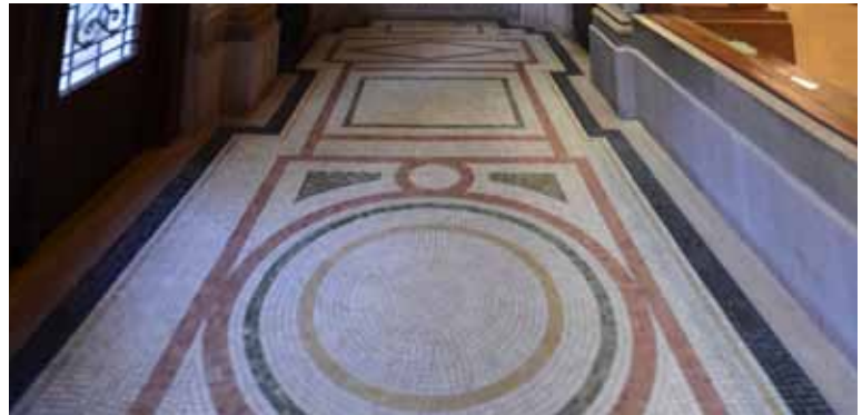
Figure 56. The original mosaic tile vestibule floor is in very good condition.
