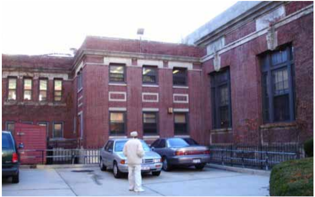
Figure 16. Rear facade from the north, ca. 2010. The Quiet Reading Room is at the upper left; the Adult Reading Room is at right. The center block includes the new elevator lobby and restrooms at the 1st floor (former staff room) and program room at the 2nd floor (former study room).
