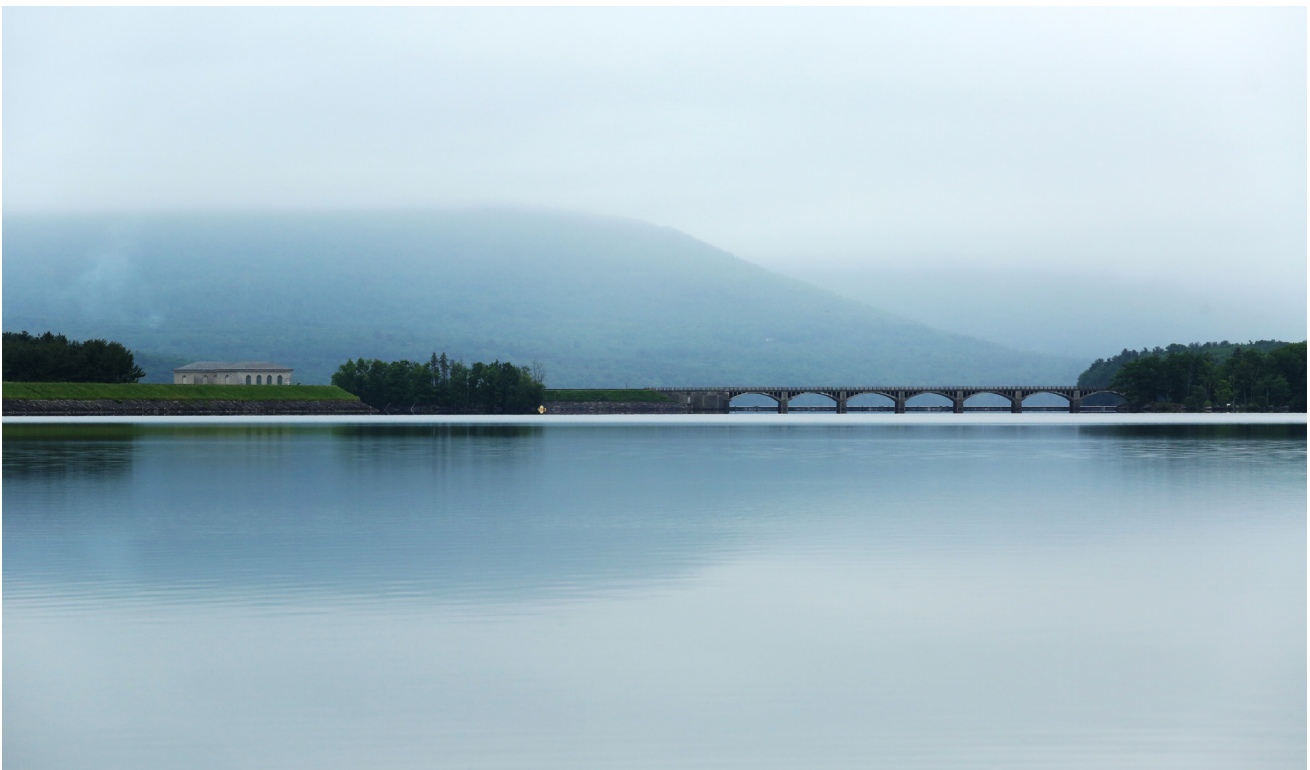
East Basin of the Ashokan Reservoir
