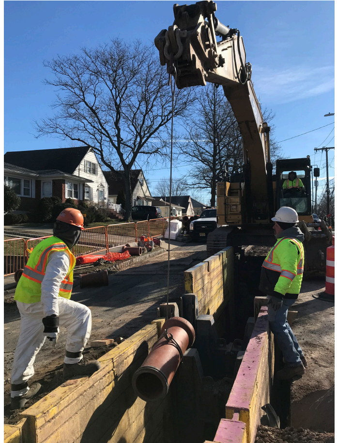
DEP Crews Working on Optimization Repairs
