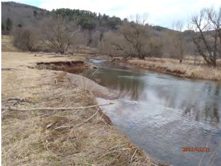
Figure 4.14. Frisbee Farm stream bank, pre-construction.
