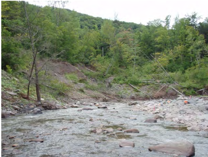
Figure 4.16. The Stony Clove Creek at Chichester reach Site 2 was the largest mapped mass failure along the creek before project construction in 2013. The mass failures were initiated more than a decade ago as the stream cut down and incised into glacial lake deposits. It was considered to be the largest chronic source of turbidity loading during non-flooding conditions.
