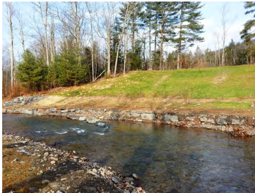
Figure 4.19. Treatment for Warner Creek Site 5 included channel realignment, in-stream rock structures, a rock terrace, and re-constructed hill slope.
