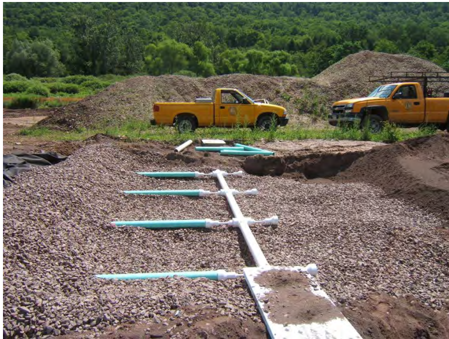
Figure 3.1. Leach field installation in Trout Creek.
