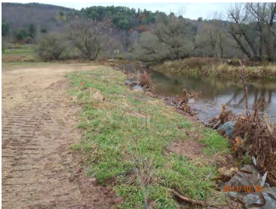
Figure 4.15. Frisbee Farm stream bank post-construction, stabilized with toe wood with live staked sod mats.
