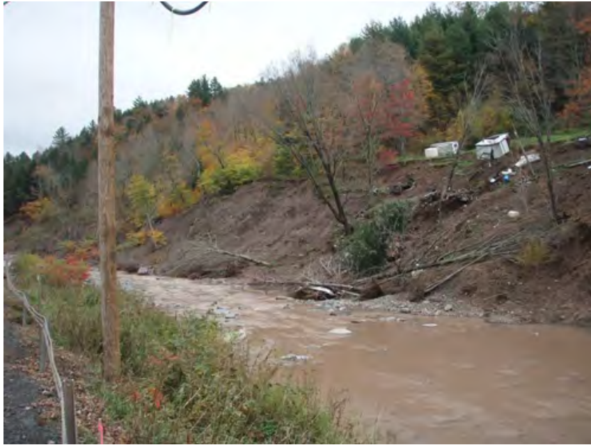
Figure 4.22. West Kill bank stabilization at NYS Route 42 prior to construction.
