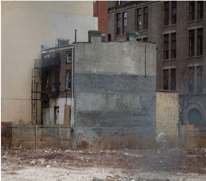
North Facade 227 Duffield Street Brooklyn Jessica Baldwin, January 2021
