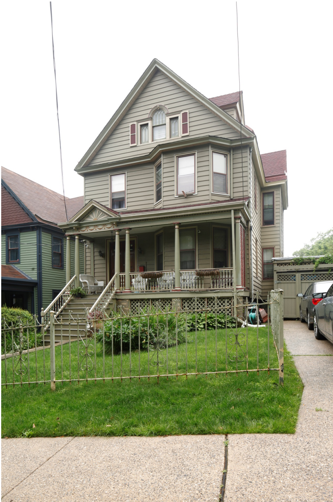
West facade, 207 St. Paul's Avenue Sarah Moses, June, 2019
