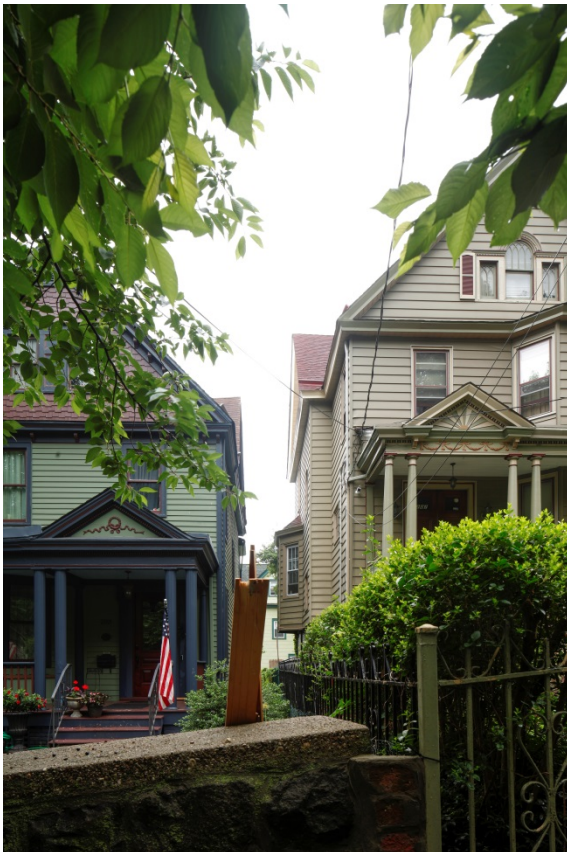
North West facade Sarah Moses June 2019
