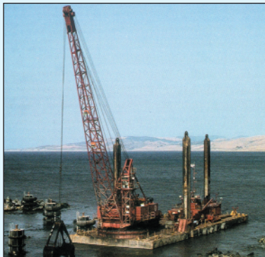
Paerdegat Basin CSO, Under Construction in Brooklyn.
