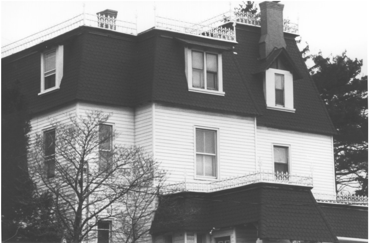
Henry Hobson Richardson House Roof and siding details
