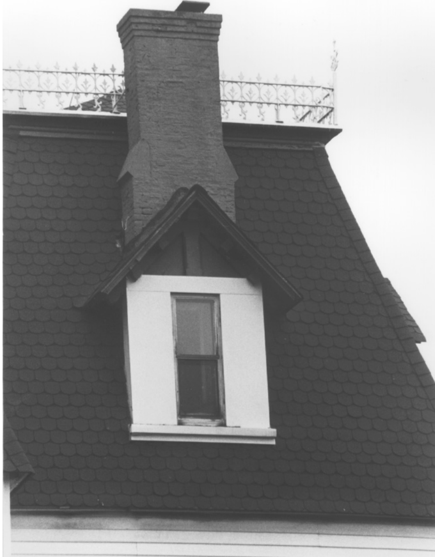
Henry Hobson Richardson House Roof and chimney details
