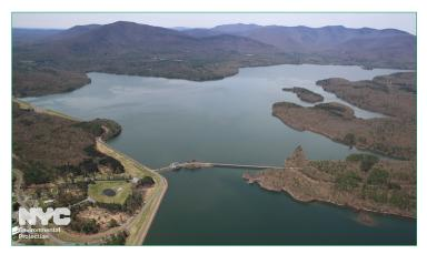
modern drainage and monitoring equipment, and the clearing of undesirable vegetation. The dam and dikes at Ashokan Reservoir total approximately 29,000 linear feet, more than the dams of all New York City's other drinking water reservoirs combined.
