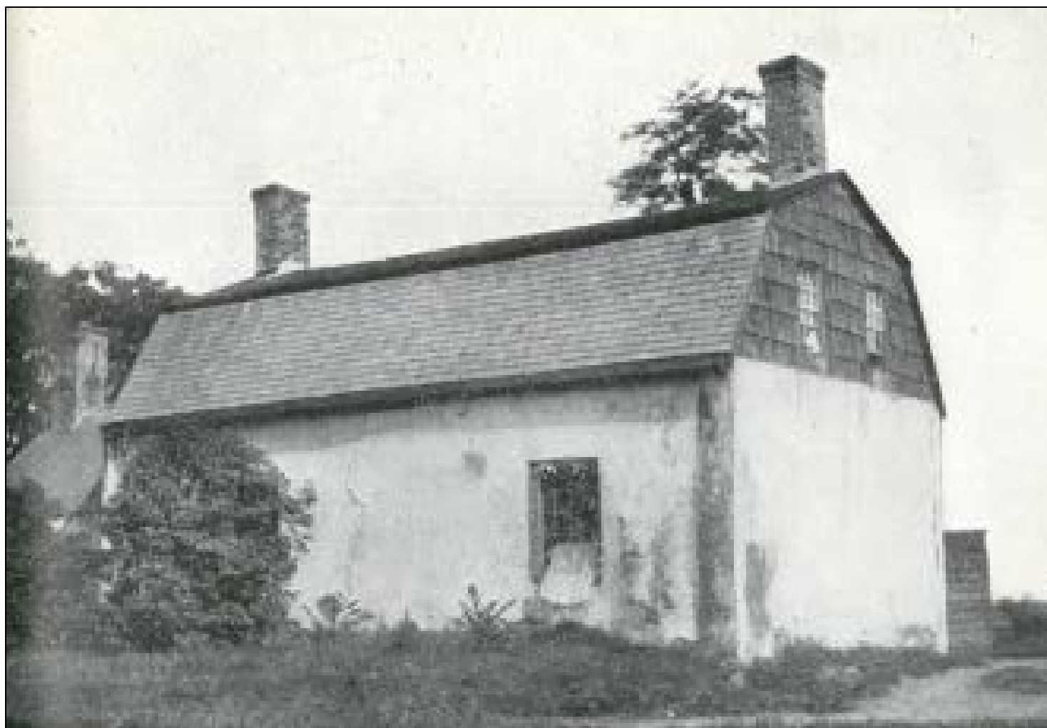
Richmond Road façade c. 1915
