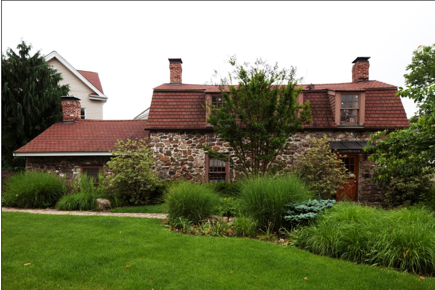
Lakeman-Cortelyou-Taylor House 2286 Richmond Road Staten Island Tax Map Block 3618, Lot 7 Photo: Christopher D. Brazee, 2014
