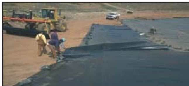
PLACEMENT OF GEOMEMBRANE
