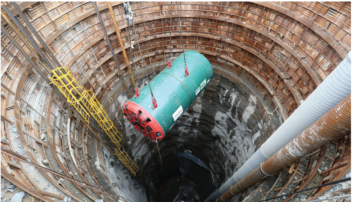
Construction of Release Works at Schoharie Reservoir
