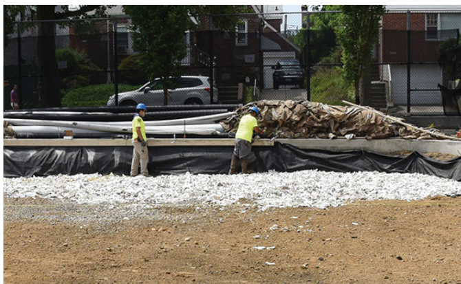
Turf field in construction
