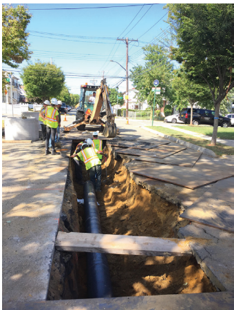
DEP crews working on a water distribution line
