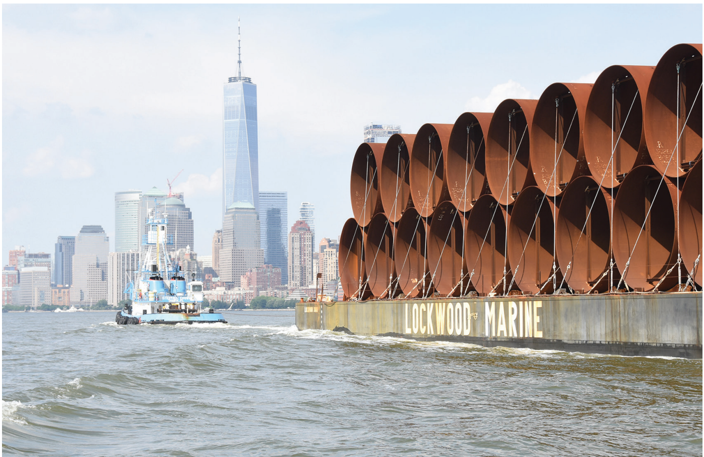
Tugboat hauling steel liners for the Delaware Aqueduct Bypass Tunnel
