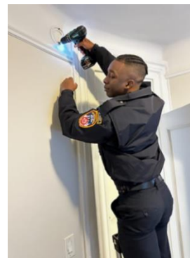
Cadet Brown installs Smoke Detector
