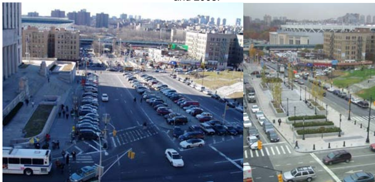
Lou Gehrig Plaza Before and After Reconstruction.
