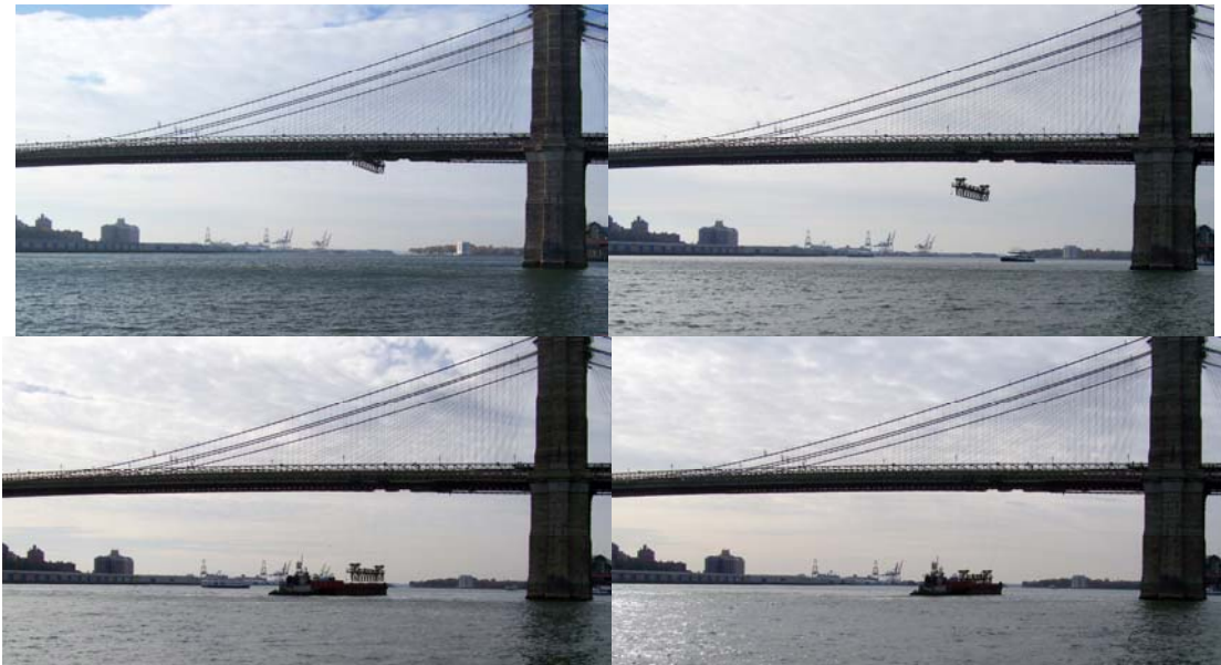
Removing the Brooklyn Bridge Main Span Travelers in 2007.
