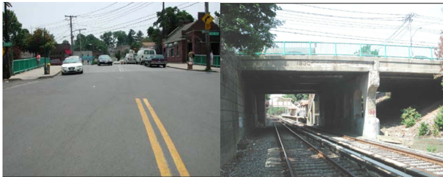
Annadale Road Bridge in 2001. (Credit: NYSDOT)
