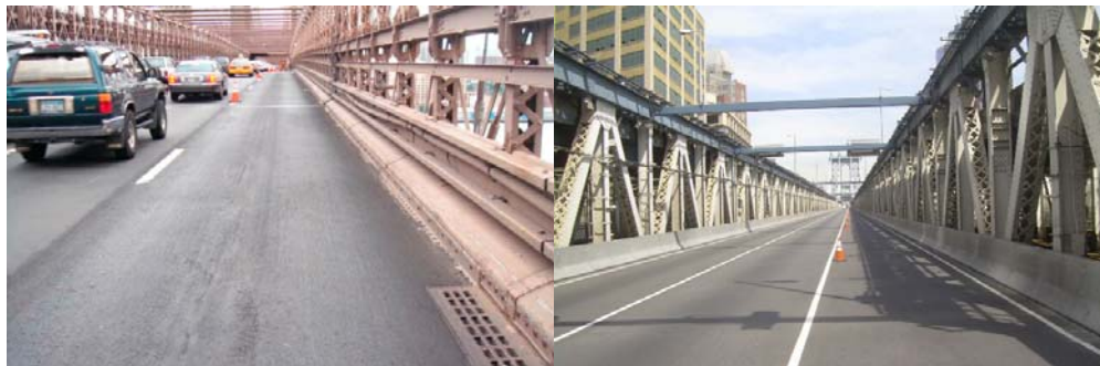
Brooklyn Bridge Wearing Surface. Manhattan Bridge Wearing Surface and Safety-Shaped Barriers. (Credit: NYSDOT)
