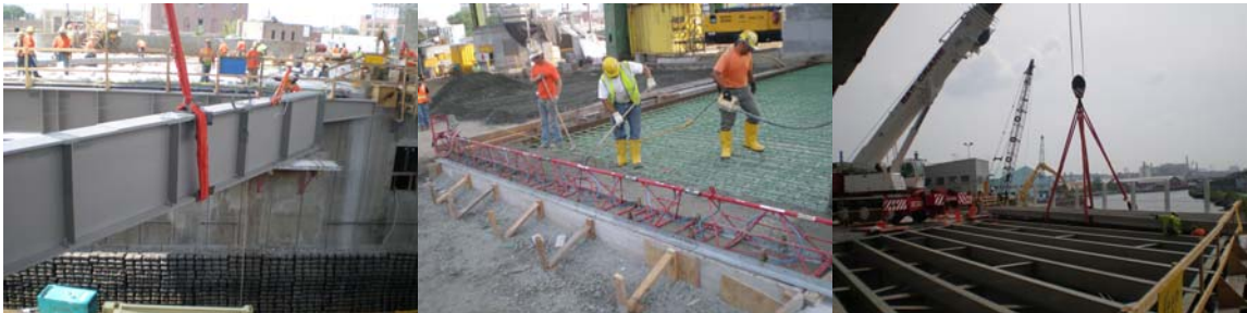
Installation of New Hamilton Avenue West Bridge Structural Steel, and Placement of Concrete for the New Northwest Sleeper Slab in July 2008. Installation of New Southwest Sidewalk in August 2008.
