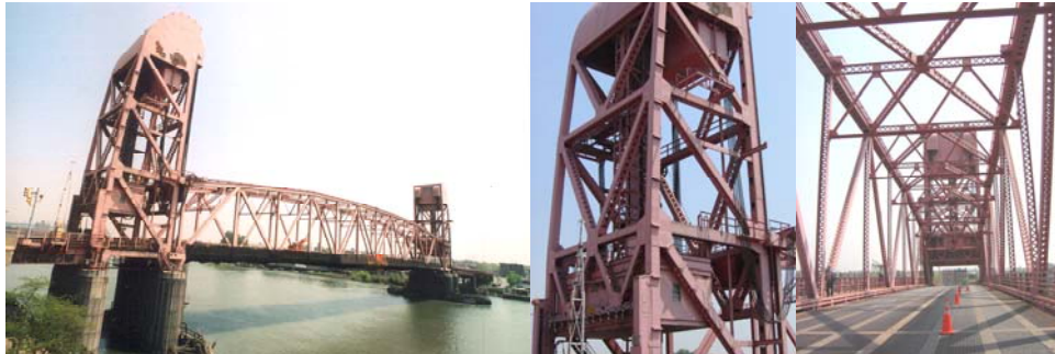
Roosevelt Island Bridge in 2005. (Credit: Peter Basich) Bridge Tower and View From Deck in 2005. (Credit: Michele N. Vulcan)
