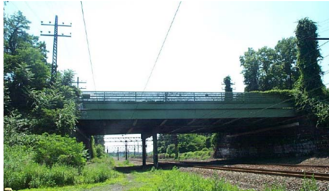
Shore Road Circle Bridge in 2003. (Credit: NYSDOT)
