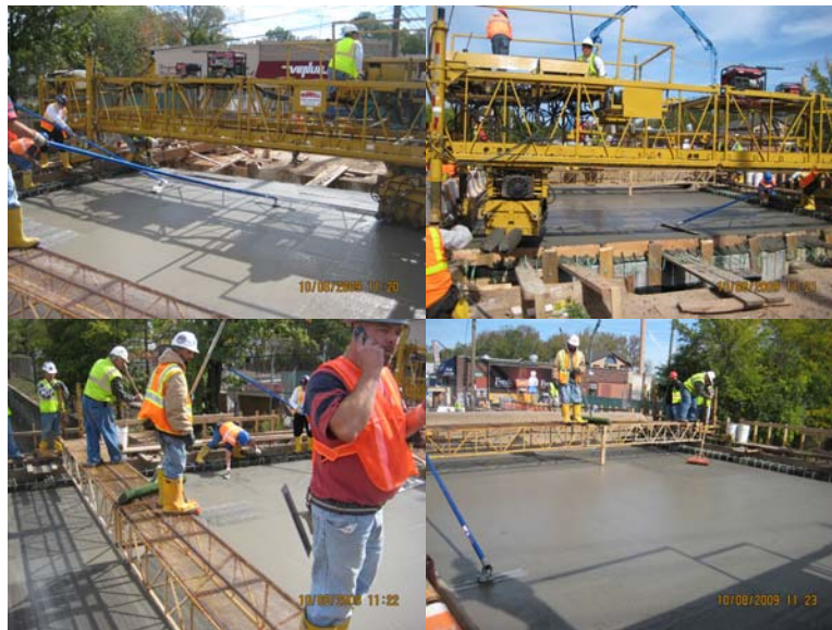
Annadale Road Bridge: Placing the Concrete Deck in October 2008.
