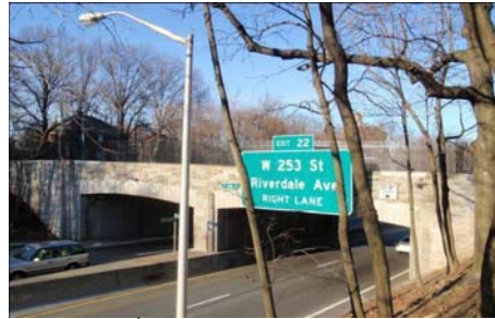
West 252 nd Street Bridge With New Signage.
