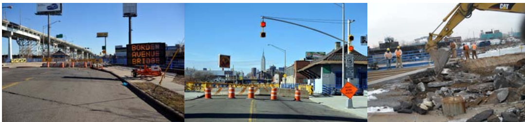
Borden Avenue Bridge Closed for Emergency Repairs in January 2009. (Credit: Bernard Ente) Roadway Excavation in January 2009.
