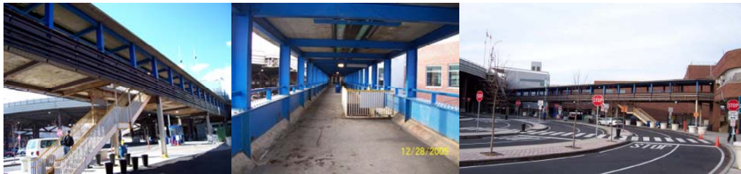
Pedestrian Breezeway - Over Commuter Drop-Off / Pick-Up Area.
