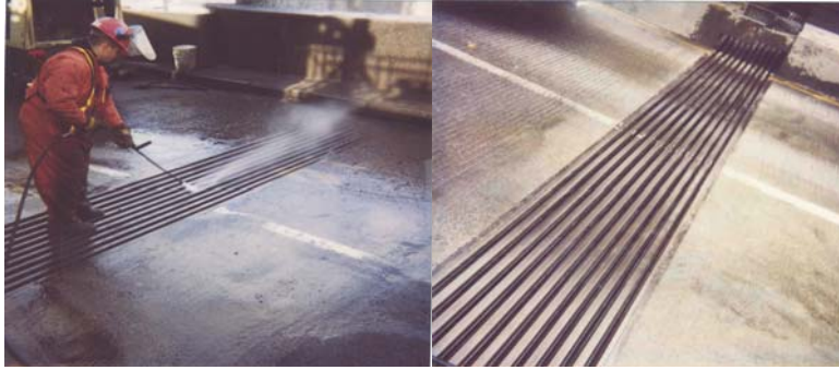
Expansion Joint Cleaning and Cleaned Joint on the Manhattan Bridge.
