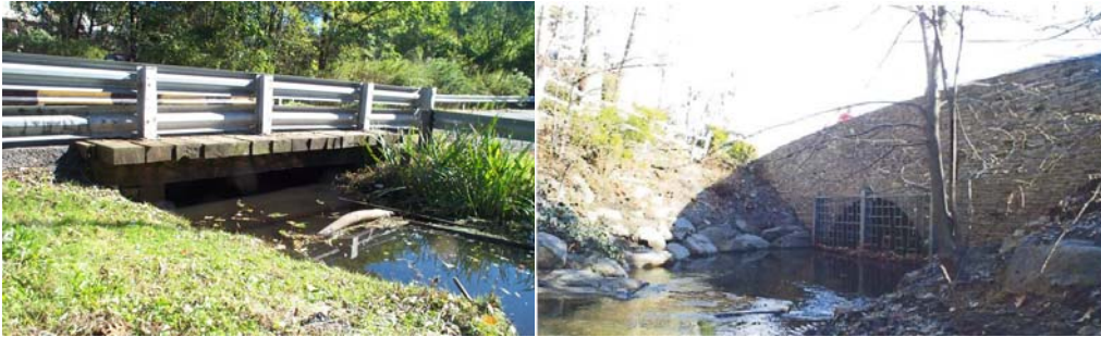
Idlease Place Culvert. Sweet Brook Road Culvert.
