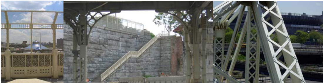
Bridge Protective Fencing and Staircase. (Credit: Michele N. Vulcan) Detail of the Bridge – Old Yankee Stadium Banner is Visible on the Right.
