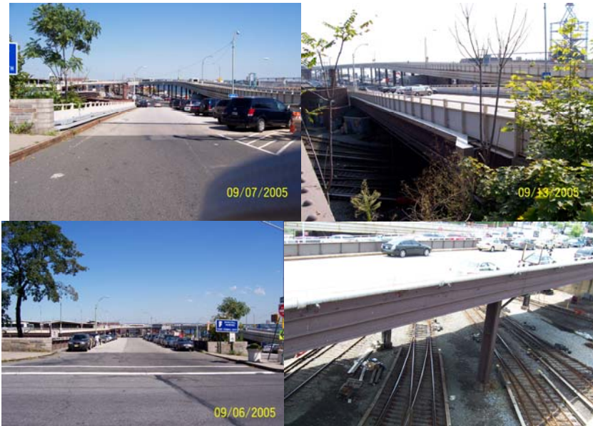
Ramp C - Commuter Entrance over SIRT Tracks. Ramp D - Commuter Exit over SIRT Tracks & Employee Parking Lot.
