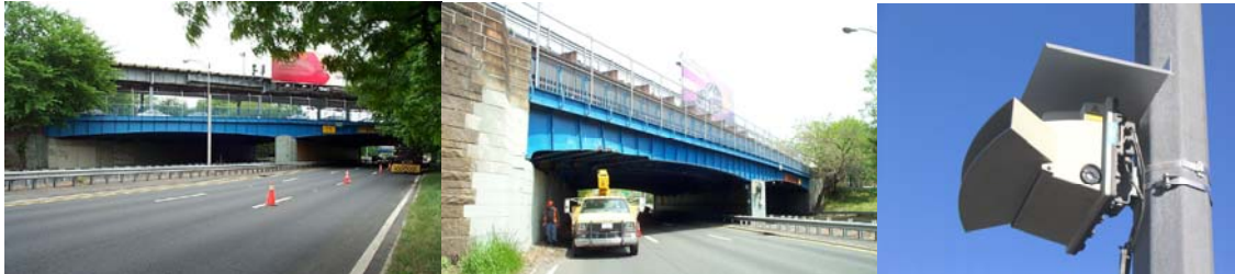
Westchester Avenue Bridge in 2001 and 2006. (Credit: NYSDOT) Overheight Sensor Unit on the Hutchinson River Parkway. (Credit: Roly Parroco)
