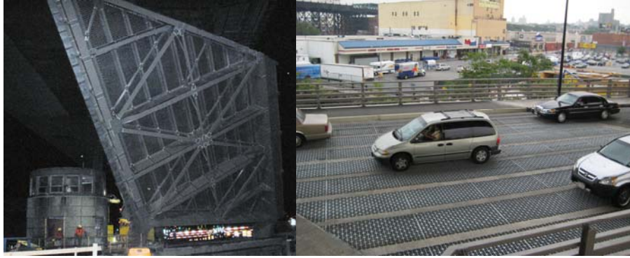
Open Manhattan-Bound Span in August 2007. Traffic on New Span.
