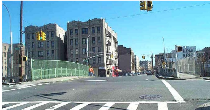
East 183 rd Street Bridge in 2002. (Credit: NYSDOT)
