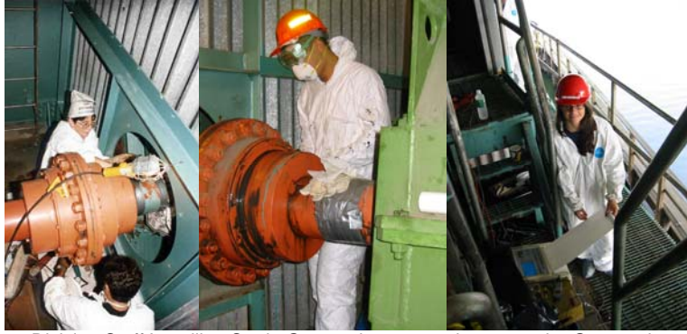
Division Staff Installing Strain Gauges in 1995 and 2006 on the Greenpoint Avenue Bridge. Checking the Measurements in 2006. (2006 Credit: Vera Ovetskaya)
