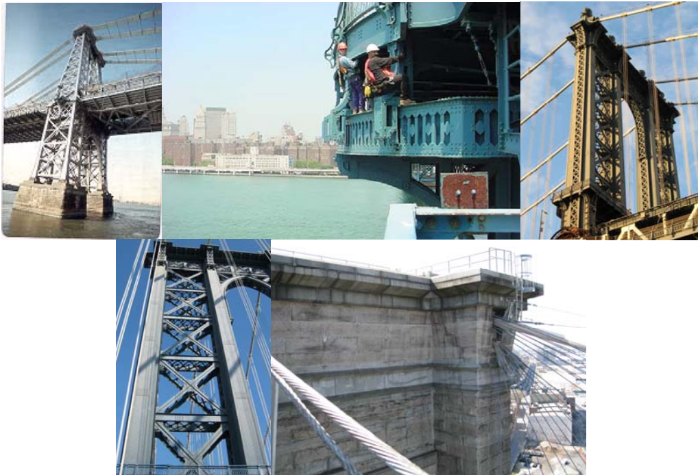
Williamsburg Bridge Tower. (Credit: Peter Basich) Inspectors on Manhattan Bridge Tower. (Inspector Credit: NYSDOT) Manhattan Bridge Tower. (Credit: Michele N. Vulcan) Manhattan Bridge Tower Detail. (Credit: Russell Holcomb) Brooklyn Bridge Brooklyn Side Tower Detail. (Credit: Jagtar Khinda)
