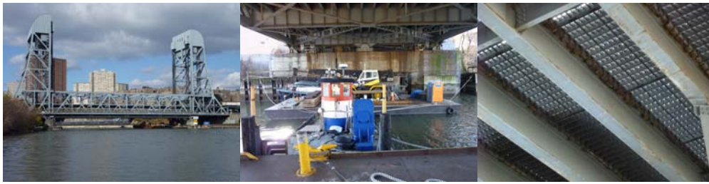
Working on the Broadway Bridge in November and December 2009.
