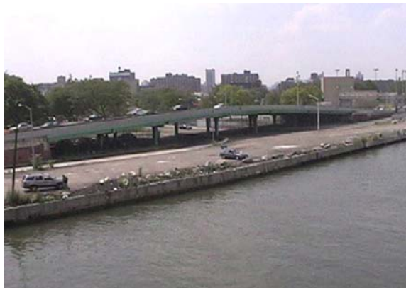
Harlem River Drive at East 127 th Street.
