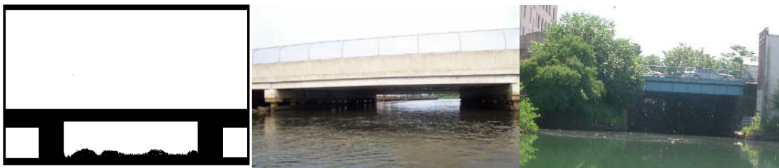
Hook Creek Bridge and Brooklyn's Third Avenue Bridge. (Credit: NYSDOT)
