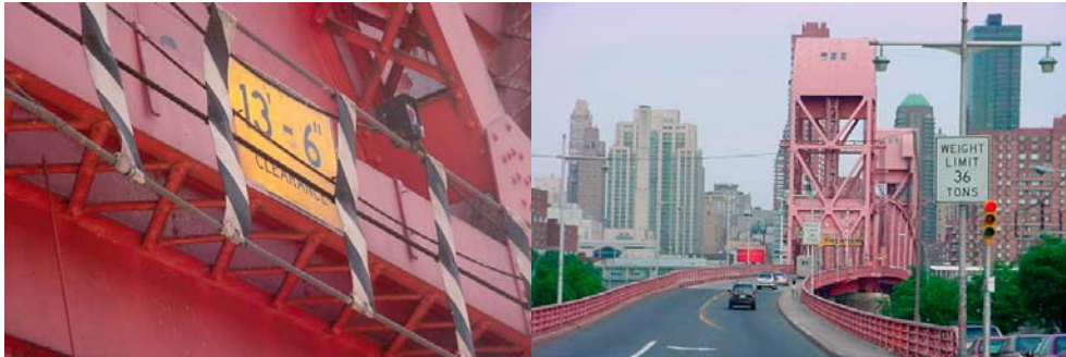
Roosevelt Island Bridge Vertical Clearance Restriction and Posted Weight Signs (Credit: NYSDOT)
