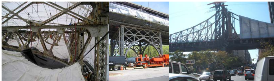
Inside the Queensboro Bridge Containment. 2005: Roadway Containment. (Roadway Credit: Michele N. Vulcan) 2006: Containment Above the Upper Roadway.
