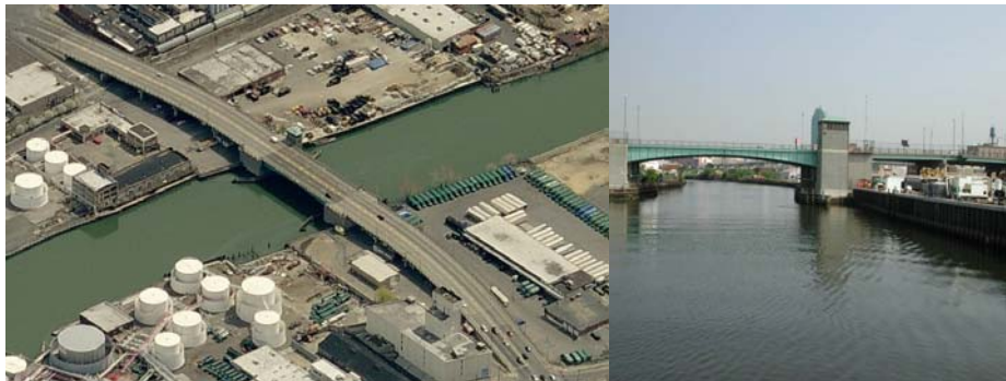
Aerial View of Greenpoint Avenue Bridge. Elevation Right Span.
