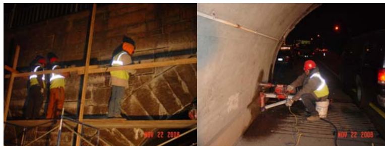
130 th Avenue Bridges: Under Deck Repair Work in November 2008.
