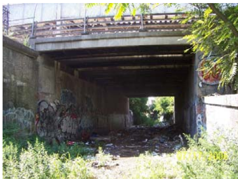
Beverly Road Bridge in 2006. (Credit: NYSDOT)
