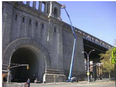
Inspecting the Exterior of the Manhattan Bridge Anchorage. (Credit: NYSDOT)
