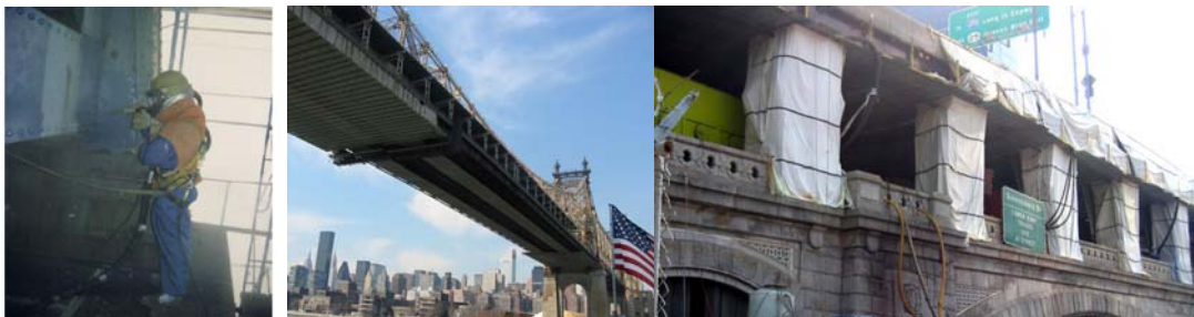
Abrasive Blasting. Platform Installed for Painting of the Queensboro Bridge (Credit: Vadim Sokolovsky) Containment on Queensboro Bridge Manhattan Ramp. (Credit: Peter Basich)
