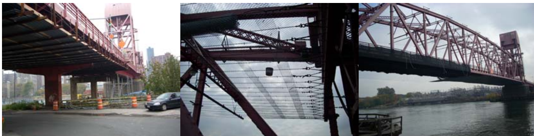
2007: Construction of the Below Deck Shield for the Queens Approach of the Roosevelt Island Bridge. Above Deck Containment on the Lift Span. The Lift Span Shield Looking Northeast.
