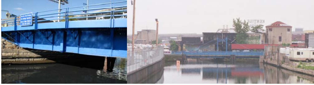
Borden Avenue Bridge. (Credit: Peter Basich). Carroll Street Bridge. (Credit: NYSDOT)
