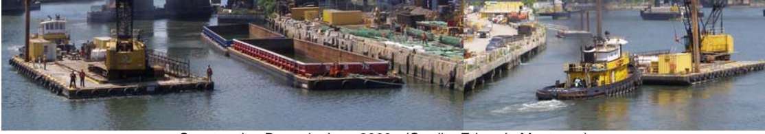
Construction Barge in June 2009. (Credit: Edgardo Montanez)
