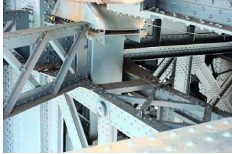
Truss Bearing on Manhattan Bridge. (Credit: NYSDOT)
