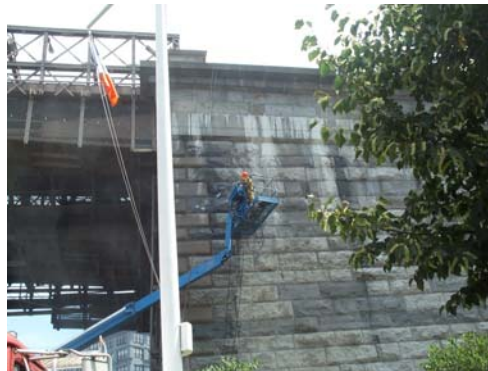
Cleaning the Brooklyn Bridge Brooklyn Anchorage in July 2007. (Credit: Serag Saad)
