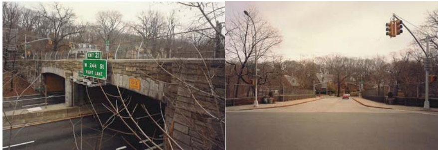
West 252 nd Street Bridge and Protective Chain Link Fence Before Reconstruction.
