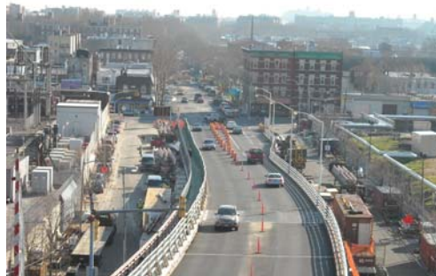
Open Queens Approach Roadway of the Roosevelt Island Bridge in December 2008.
