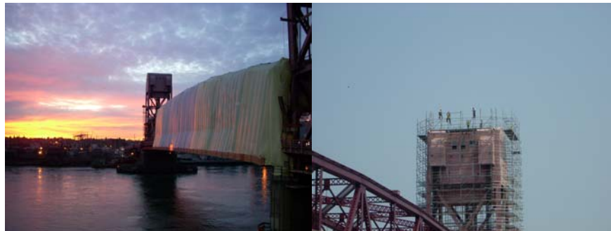
Lead Paint Removal Containment on the Roosevelt Island Bridge Lift Span in January 2008. Scaffolding Erection on the East Tower in July 2008.
