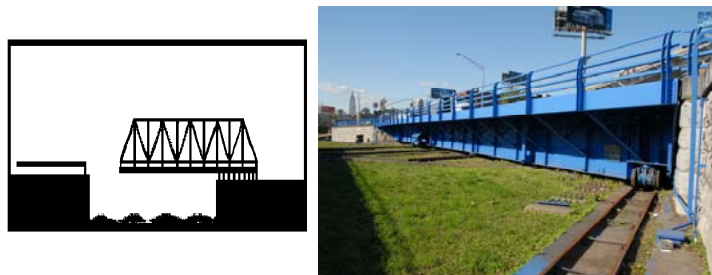
Borden Avenue Bridge. (Credit: Peter Basich).
