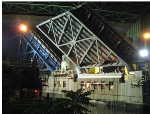
Open Hamilton Avenue Bridge in August 2007.
