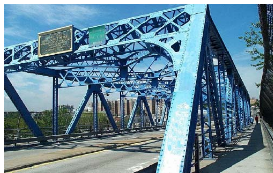
East 174 th Street Truss Bridge over Sheridan Expressway. (Credit: NYSDOT)
