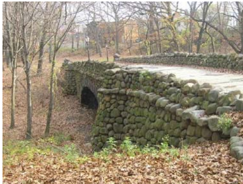
Highland Park Bridge. (Credit: NYSDOT)
