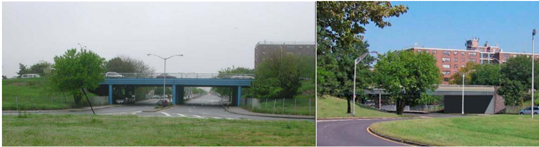
Rockaway Parkway Bridge in 2002. (Credit: NYSDOT) Proposed Rockaway Parkway Bridge.
