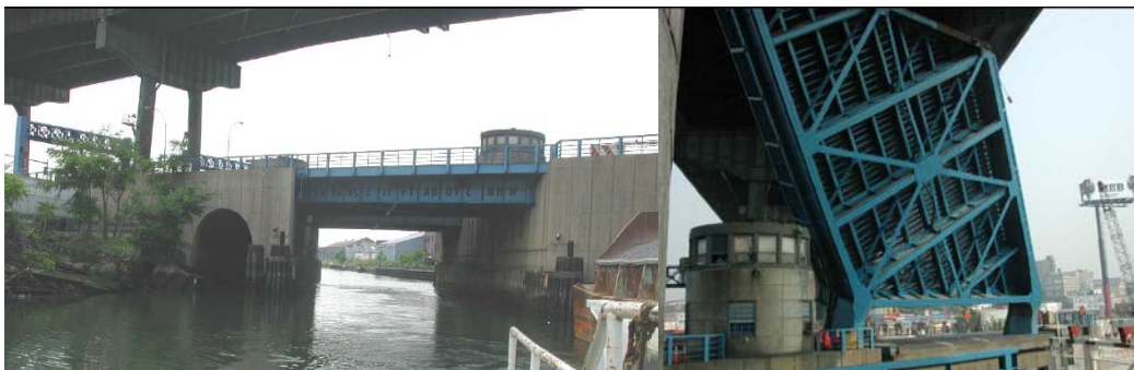
Old Hamilton Avenue Bridge. (Credit: NYSDOT)
