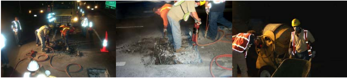
2005: Masonry Crews and Highway Repairers Repairing Recurrent Potholes on the Eastbound Brooklyn-Queens Expressway, Just Past the Middagh Street Underpass. Break-Out and Removal of the Old Asphalt Roadway and Concrete Deck. Installing New Concrete With Rebar in the Cutout on the Eastbound BQE. (Credit: Anthony Napolitano)
