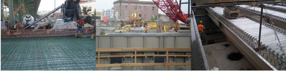
Placement of New Concrete on the Hamilton Avenue Southwest Approach Slab, Installation of New West Bridge Structural Steel, and Installation of New West Bridge Deck and Counterweight in July 2008.
