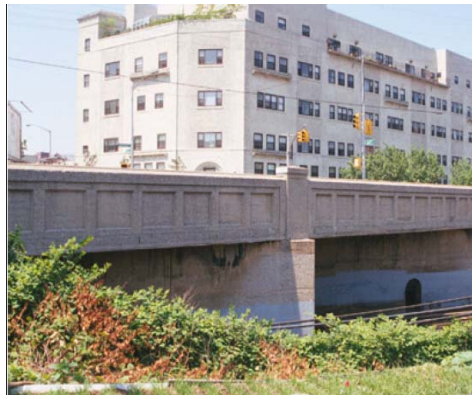
Woodside Avenue Bridge. (Credit: NYSDOT)
