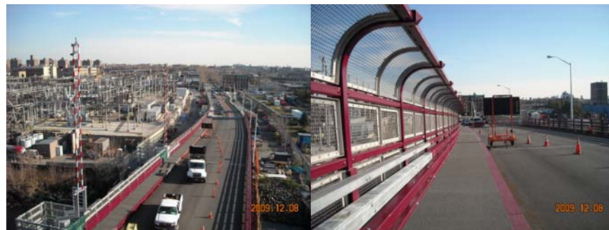
December 2008: East Approach Roadway and Sidewalk.
