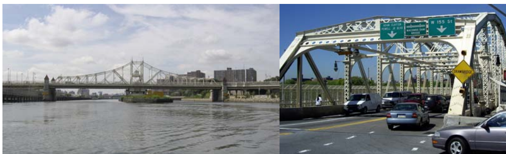
Macombs Dam Bridge (Elevation Credit: NYSDOT).
