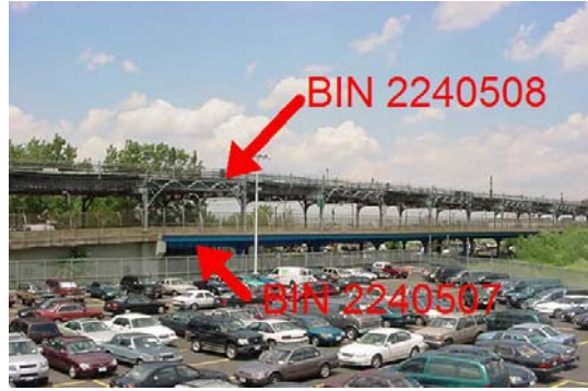
Roosevelt Avenue Bridge (#2240507) in 2002. (Credit: NYSDOT)
