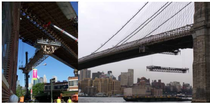
Lifting Traveler #4 in June 2008. Lifting the New Manhattan Main Span Traveler to the Underside of the Bridge on November. 20, 2008. (Main Span Credit: Bojidar Yanev)
