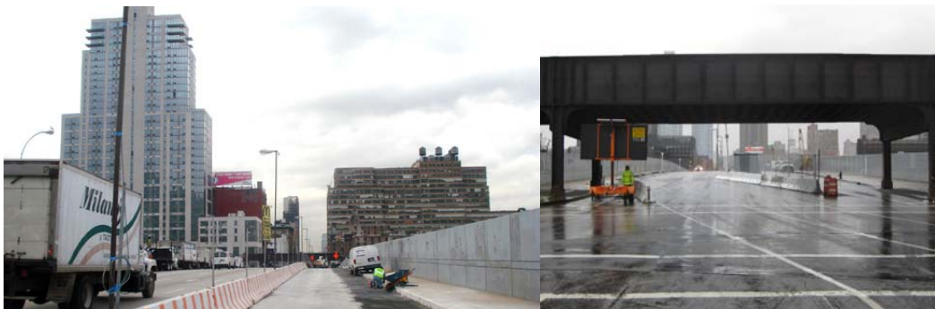
11 th Avenue Viaduct Stage 1A Construction. Traffic Enforcement Agent on Duty During Stage 1B Construction.
