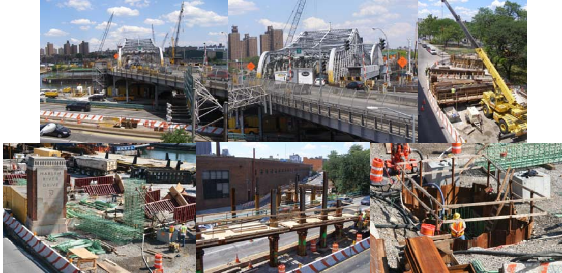
Current Willis Avenue Bridge and Construction Site in July 2008.
