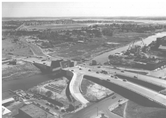
Unionport Bridge in 1953.
