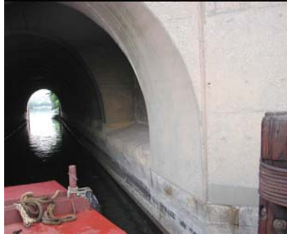
Hamilton Avenue Bridge Abutment. (Credit: NYSDOT)
