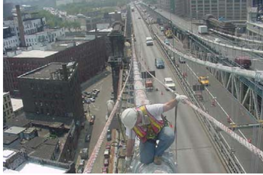
Inspector on Manhattan Bridge Cable. (Credit: NYSDOT)
