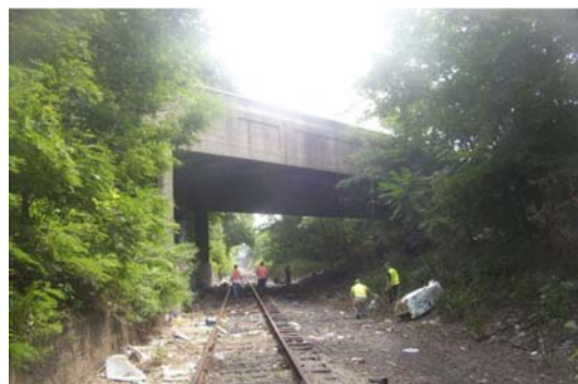
50 th Street Bridge in 2003. (Credit: NYSDOT)
