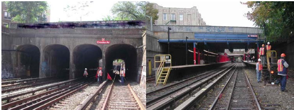
Crooke & Newkirk Avenue Bridges. (Credit: NYSDOT)
