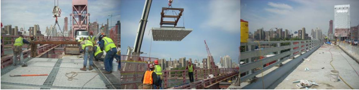
Concrete Filled Grid Deck of the Queens Approach in April and May 2008. Stage I Roadway Construction of the Queens Approach in July 2008.
