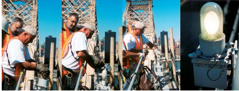
Changing a Bulb on the Queensboro Bridge Necklace Lighting. (Credit: Peter Basich)
