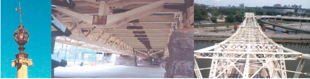
2000 – 2002: John Hooper Fountain Globe. New Trusses at the Jerome Avenue Approach to the Bridge. View of the Roadway in 2004 From Above the Control House – Old Yankee Stadium is on the Right. (Roadway Credit: Peter Basich)
