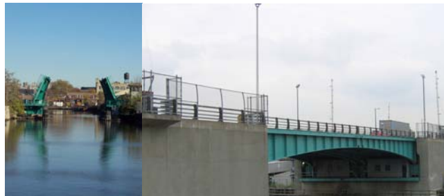
Union Street Bridge. Greenpoint Avenue Bridge. (Greenpoint Credit: Michele N. Vulcan)
