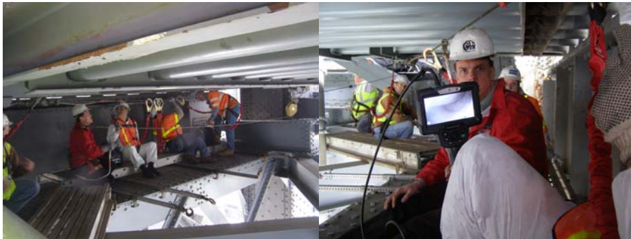
Director of Bridge Management Kevin McAnulty (in Red Jacket) Utilizing a BoreScope to Inspect the Joints of the Williamsburg Bridge in April 2009.
