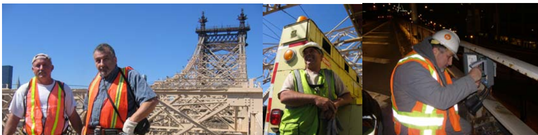
Electrician Robert Stackpole and Supervisor Electrician Ben Cipriano Atop the Queensboro Bridge. Electrician Helper Richard Parisi. (Credit: Peter Basich) Supervisor Electrician Ben Cipriano Installing an Outlet on the Brooklyn Bridge. (Credit: Hany Soliman)
