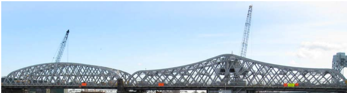
Willis Avenue Bridge. (Credit: Brain Gill)
