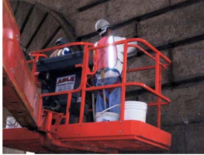
Pointing Joints on the East Face of the Brooklyn Anchorage of the Manhattan Bridge.
