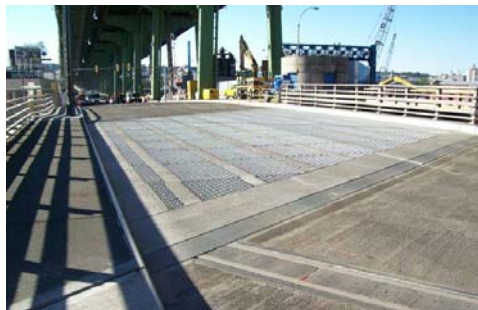
Hamilton Avenue Bridge Deck. (Credit: NYSDOT)
