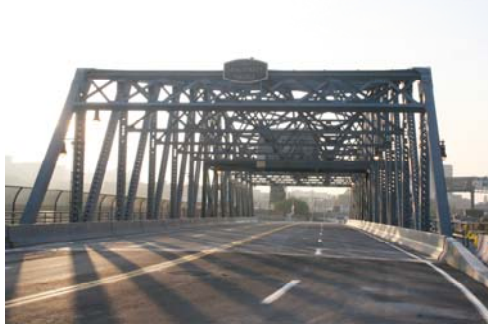
2007: New Bridge Ready for Traffic.
