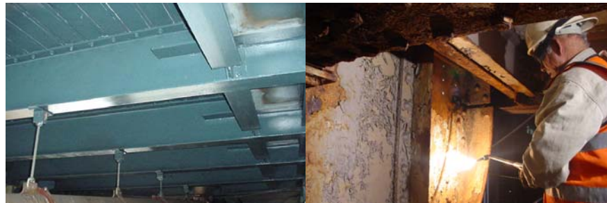
Stringers on the Manhattan Bridge. (Credit: NYSDOT) Bridge Repairer & Riveter Joseph Antony Repairing a Red-Flagged Stringer on the Bridge. (Credit: Hany Soliman)
