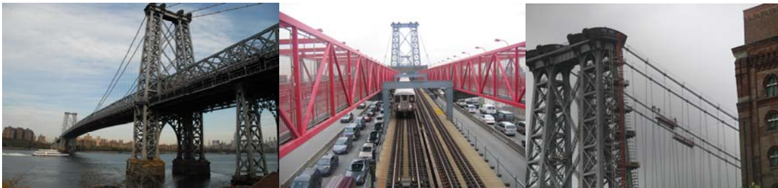
Williamsburg Bridge. Bridge Subway Structure. (Credit: Peter Basich). Contract #: Looking South at a Cable Band Retensioning Crew.
