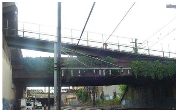
Bryant Avenue Bridge in 2002. (Credit: NYSDOT)
