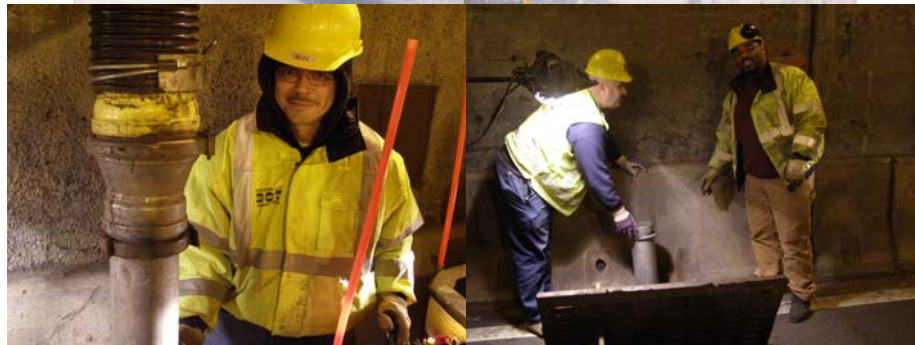
Cleaning Catch Basins on the Manhattan Bridge. Drain Crew: Highway Repairer Anthony Irizarry, Supervisor Highway repairer Michael Parise, and Assistant City Highway Repairer Giovanni Caballero. (Crew Credit: James Campbell)
