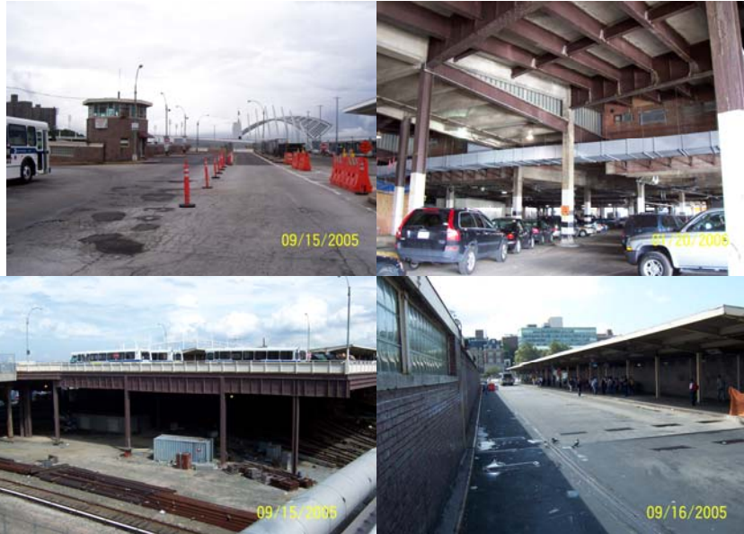
Bus Station North - over Terminal Building, SIRT Station and Employee Parking Lot. Station South - over SIRT Station and Employee Parking Lot.
