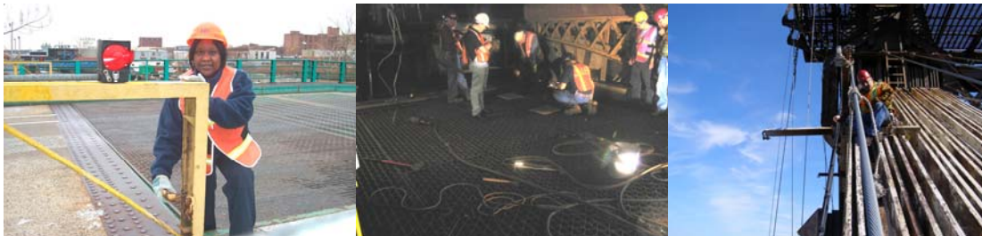
Bridge Operator Mary Harrigan at the Union Street Bridge. (Credit: Adal Maldonado) Bridge Repairer/Riveters Repairing the Willis Avenue Bridge Grating. (Credit: Reza Taheri) Supervisor Electrician Ben Cipriano Repairing a Damaged Electrical Cable on The Queensboro Bridge in March 2007. (Credit: Bala Nair)
