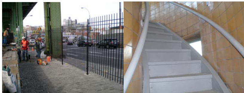
Installation of New Hamilton Avenue Parking Fence at the North Median Area in November 2008. Painting the Existing Control House Staircase in December 2008.
