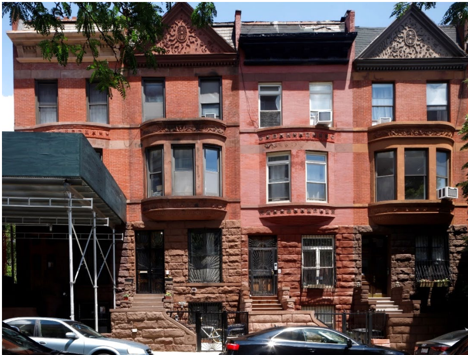
Figure 2 Houses in the row from 305-321 West 136th Street Jessica Baldwin, LPC, 2021
