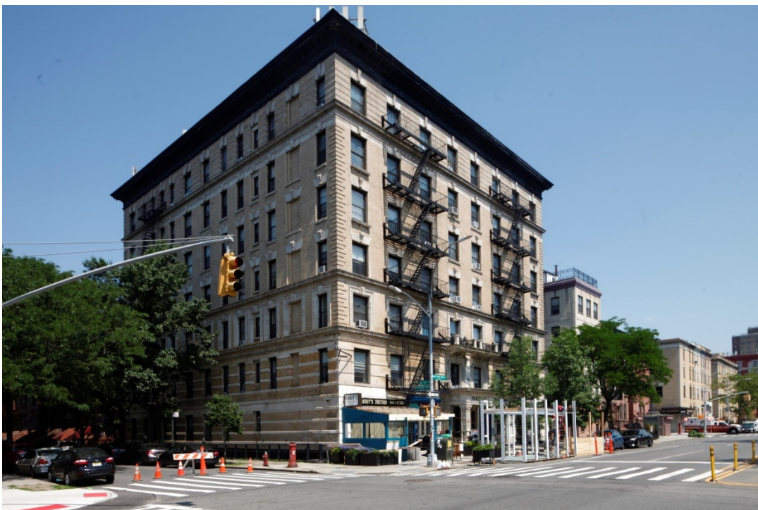
Figure 6 The Rangeley Apartments, 2340-2344 Adam Clayton Powell Jr. Boulevard Jessica Baldwin, LPC, 2021
